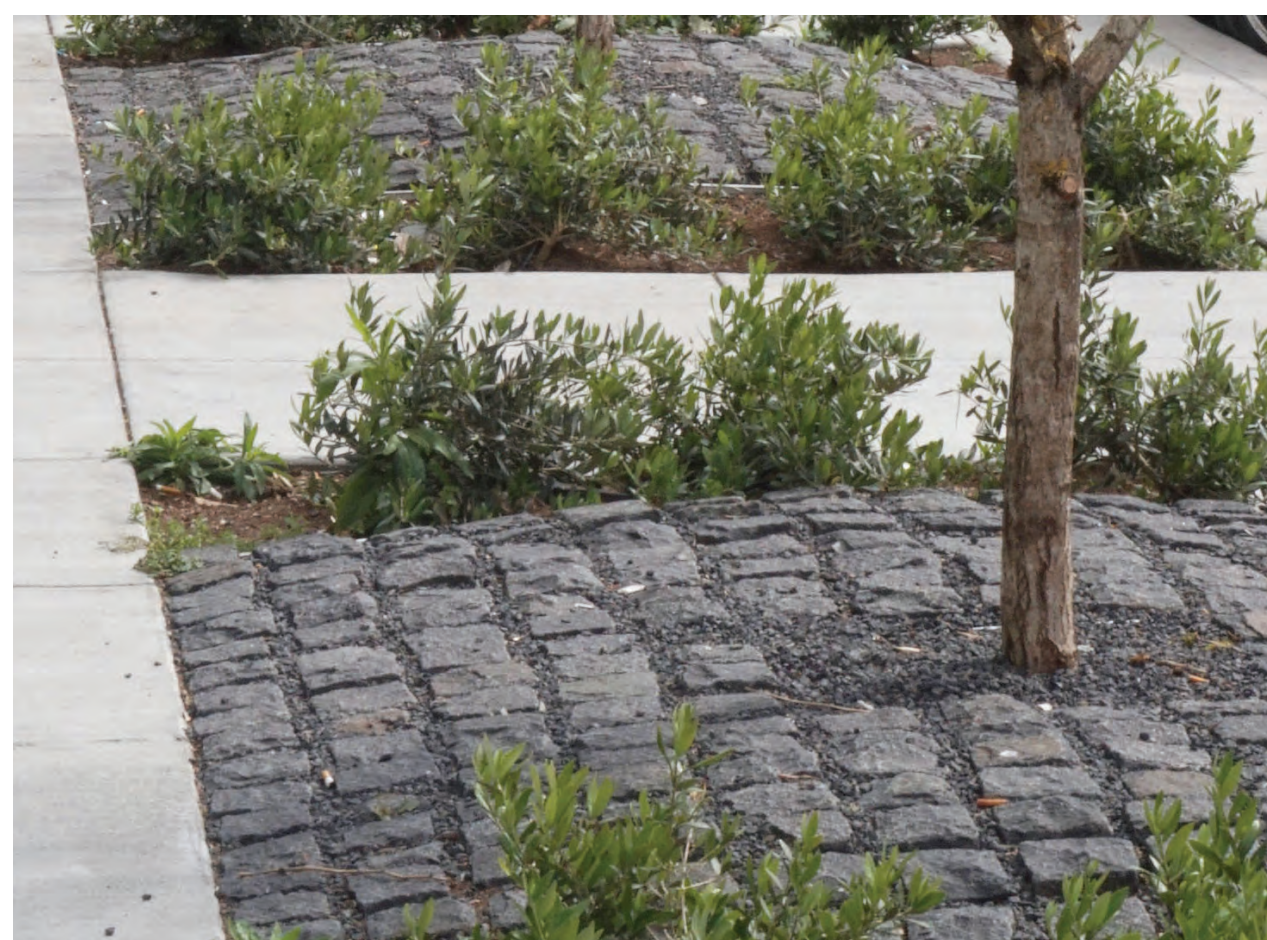
STONE COBBLES AT TREE WELLS
