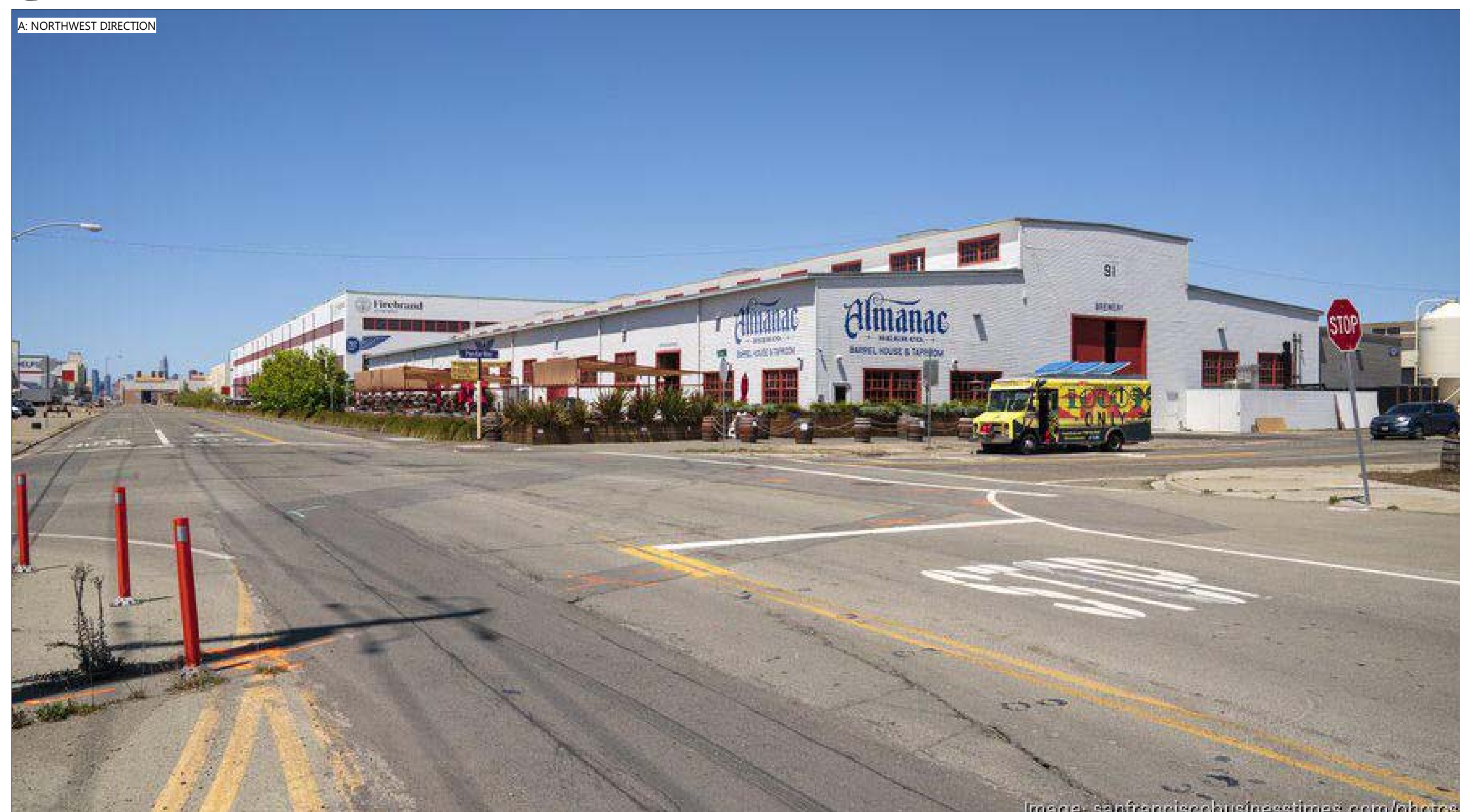
3 INTERSECTION AT PAN AM WAY AND W TOWER AVE
