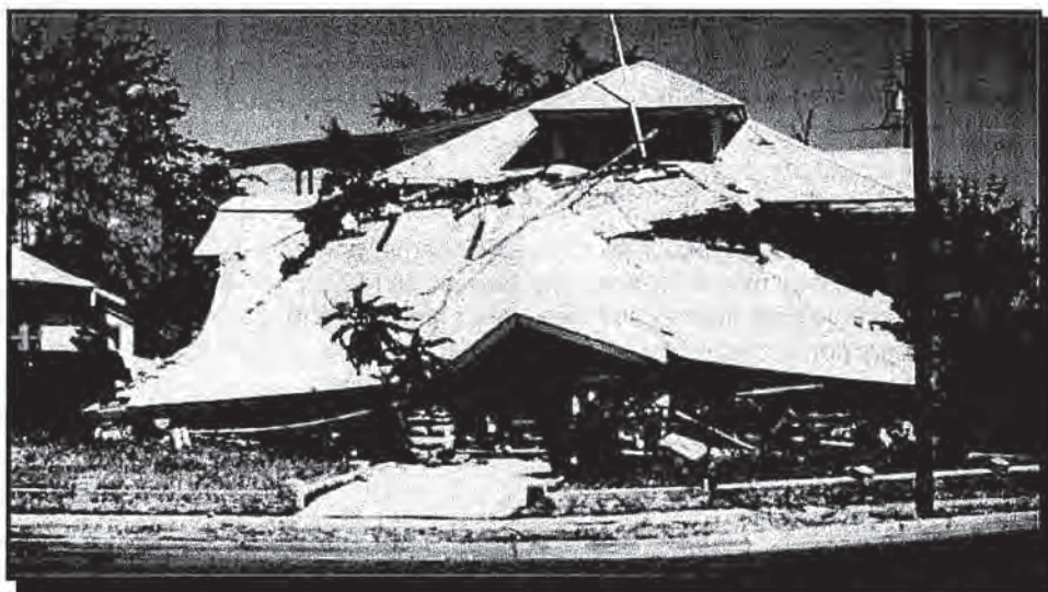
Additional damage from aftershocks
