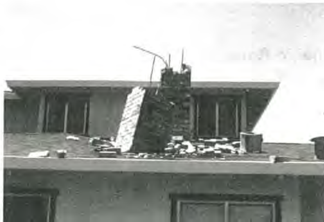
Figure 34 - Morgan Hill Earthquake. Broken chimney fell on roof.
