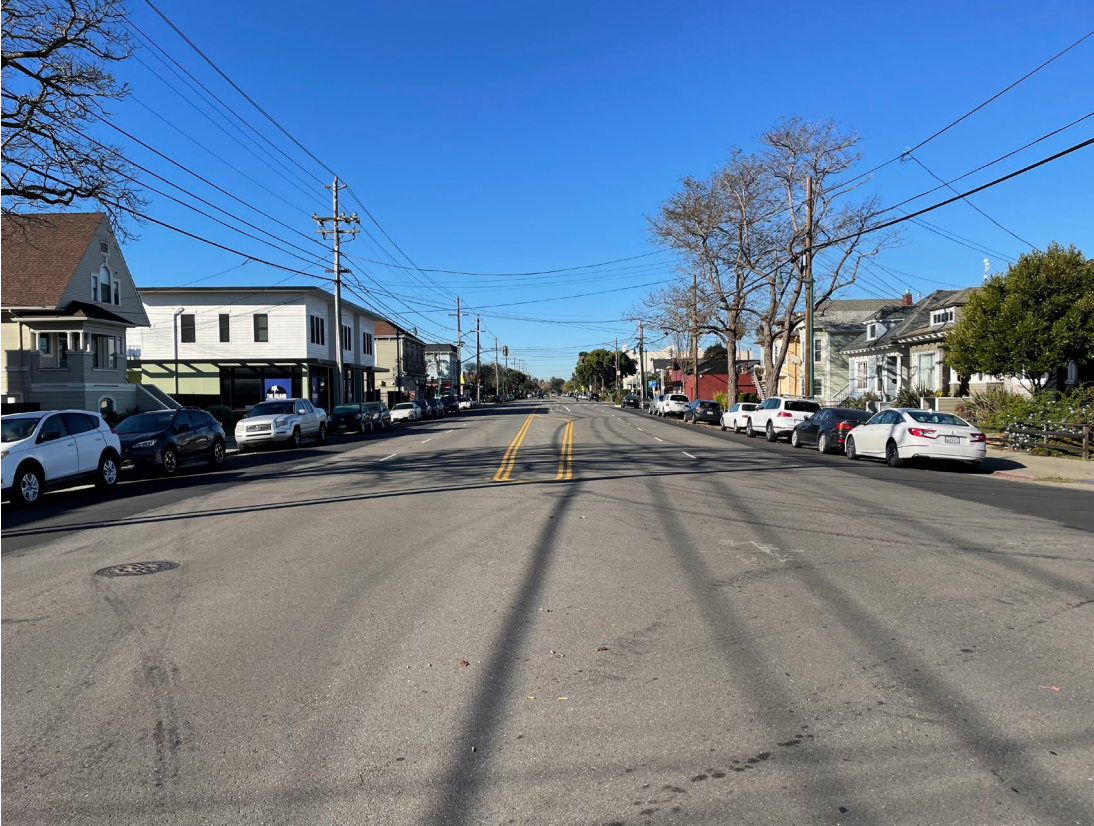
Looking East at Lincoln Ave. / Concordia St.
