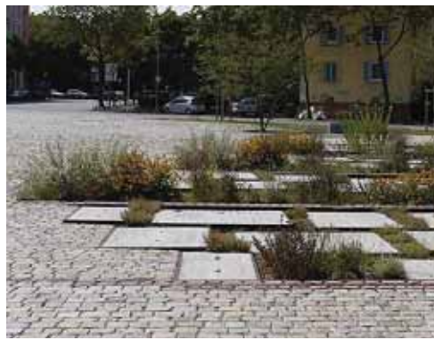
"Eroding" Stormwater Treatment Area
