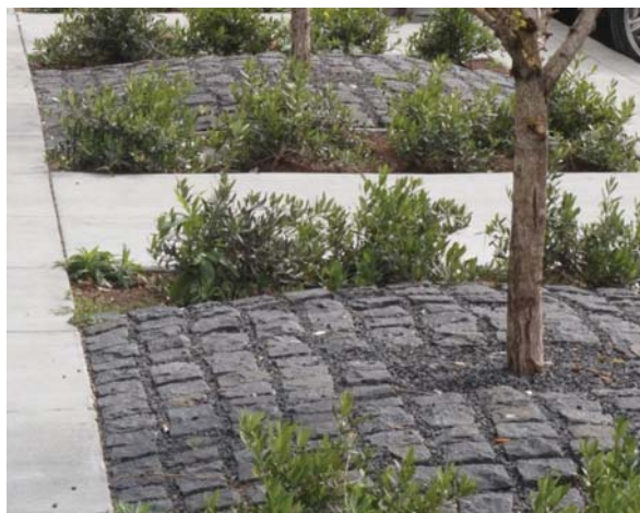
STONE COBBLES AT TREE WELLS
