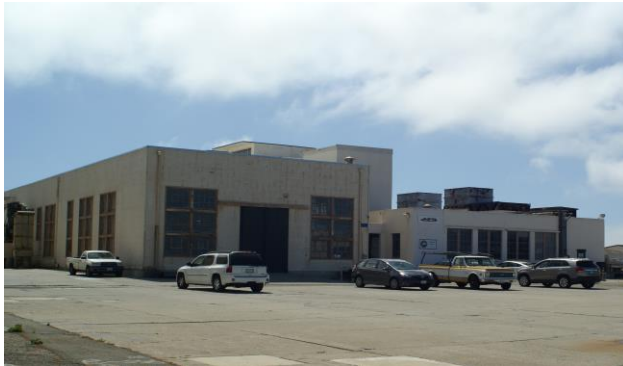
Figure 19. Building 14, facing southeast.
