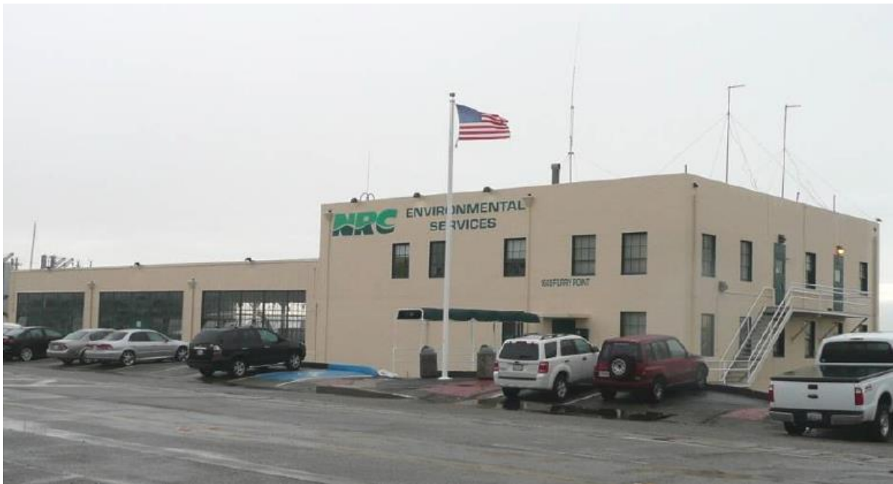
Figure 14. Building 15, primary façade, facing northwest. Source: JRP Consulting
