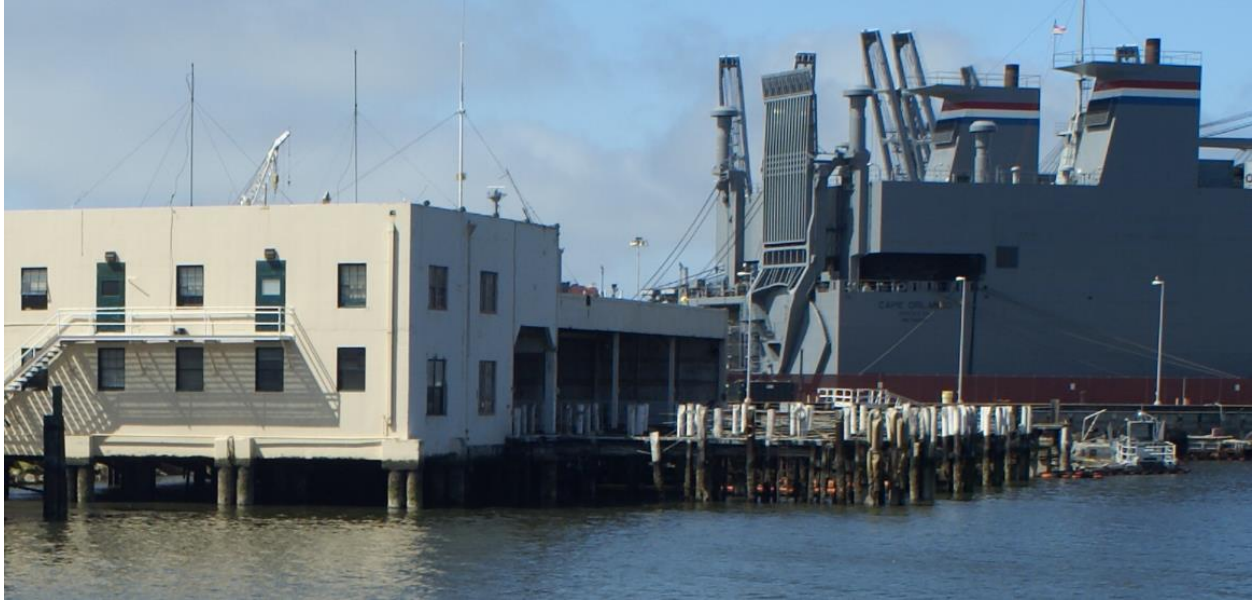
Figure 15. Building 15, side and rear facades, facing west.
