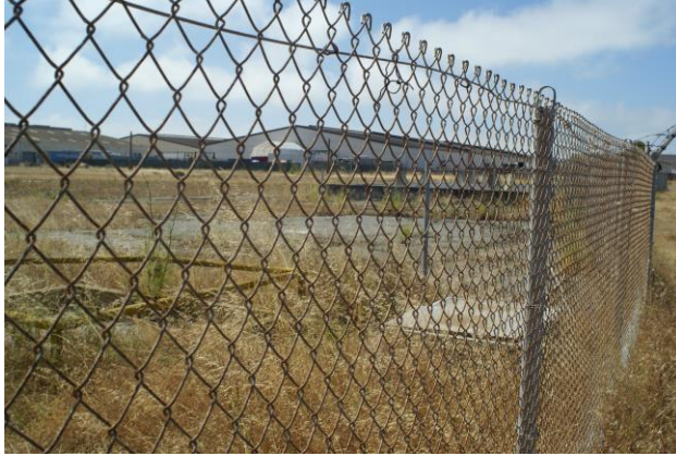
Figure 10. Chain link fence enclosure, facing southeast.
