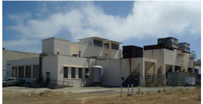
Figure 20. Building 14, facing northeast.
