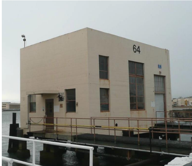
Figure 16. Building 64, primary and southwest facades, facing northeast. Source: JRP Consulting
