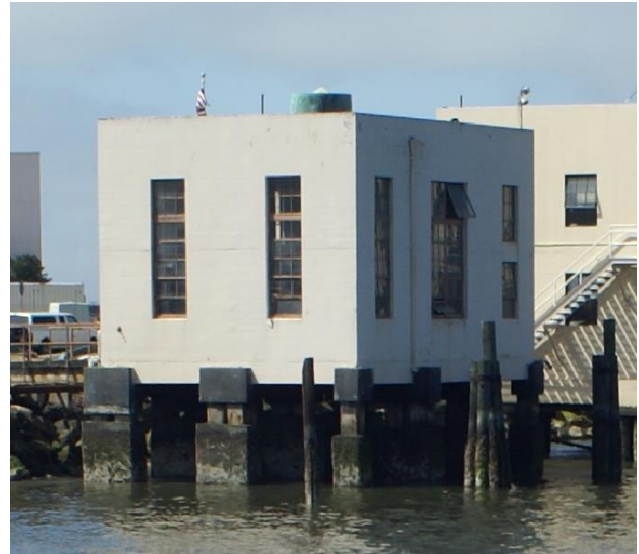
Figure 17. Building 64, northeast and rear facades, facing west.
