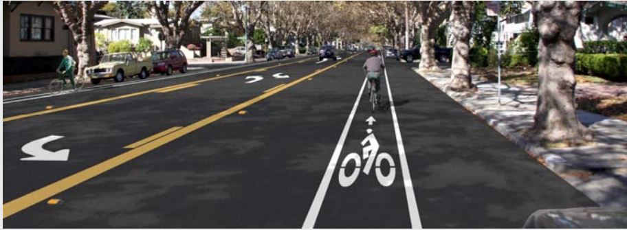
Central Avenue Safety Improvement Project
