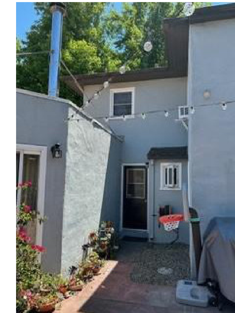
BACK OF HOUSE FROM NORTH
