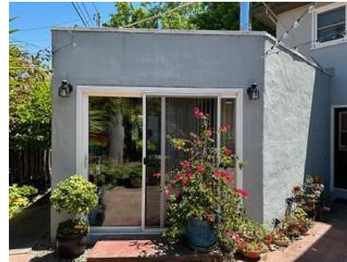
ADDITION TO BE REMOVED - FROM NORTH
