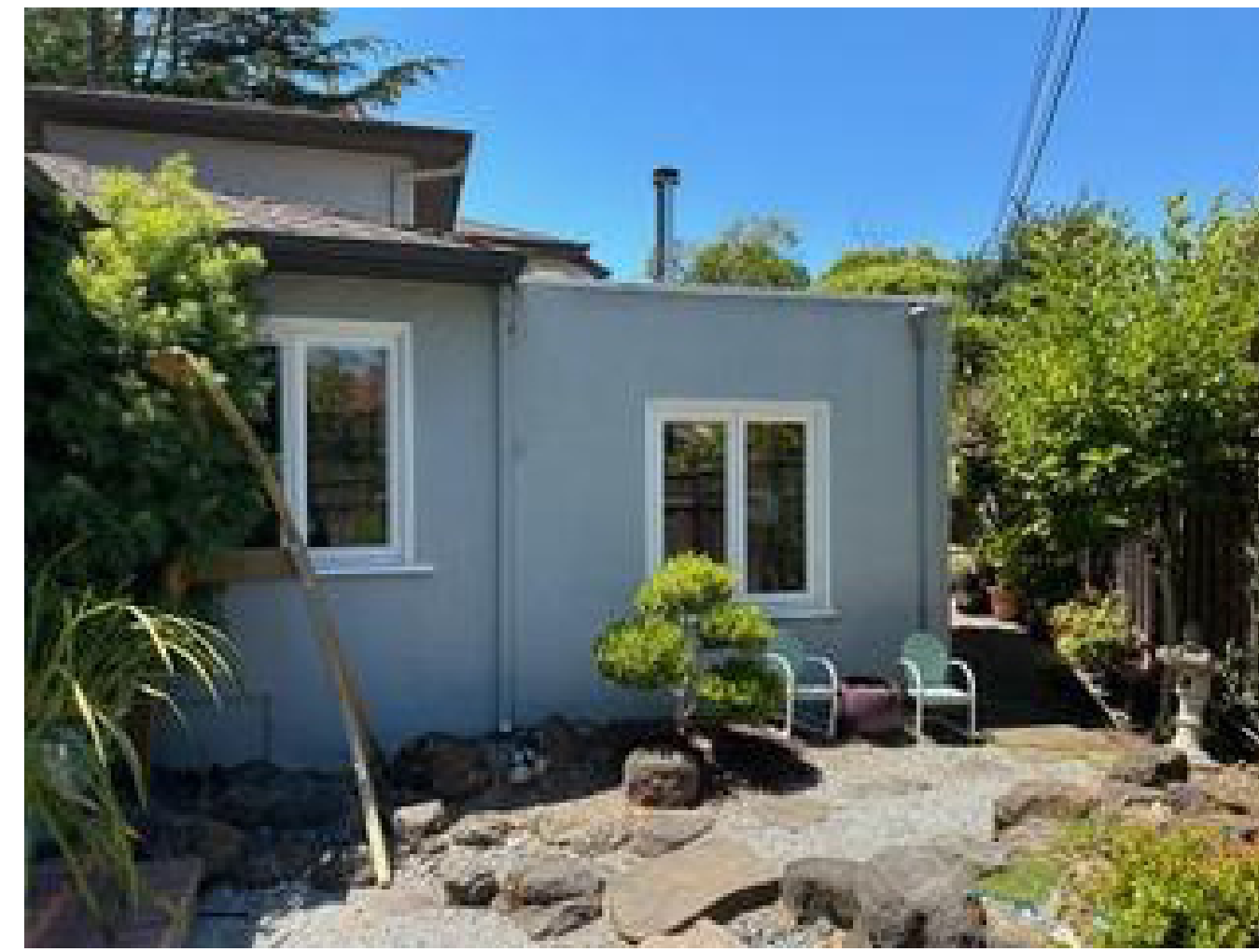
NORTH ADDITION TO BE REMOVED - FROM EAST
