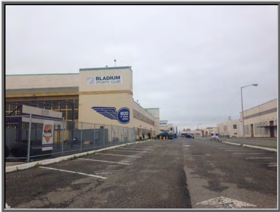
North Side of Subject Building
