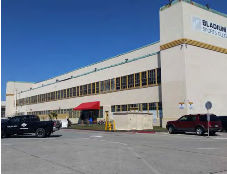
Subject view northwest from parking lot
