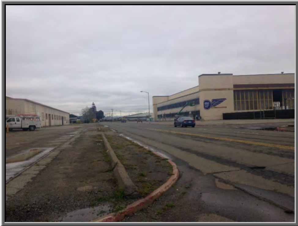
W. Tower Avenue Looking East
