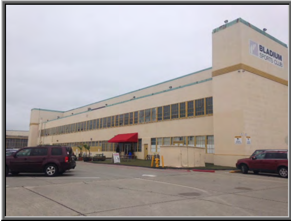
South Side of Subject Building
