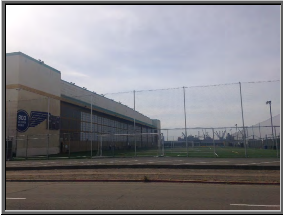
West Side of Subject Building
