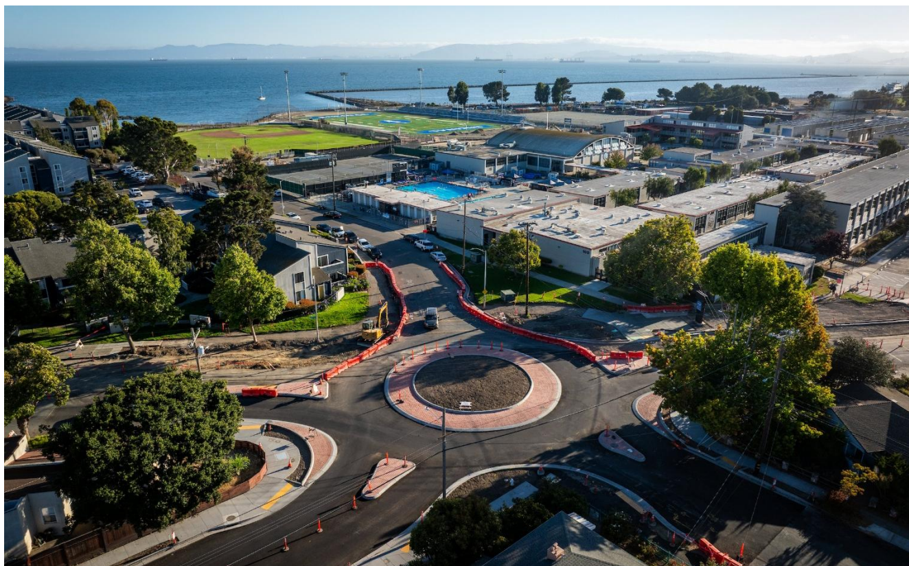
Central Avenue under construction in 2025. Photo by Maurice Ramirez.
