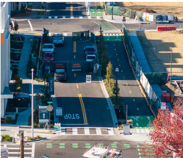
Cross Alameda Trail segment under construction along Clement Avenue. Photo by Maurice Ramirez.
