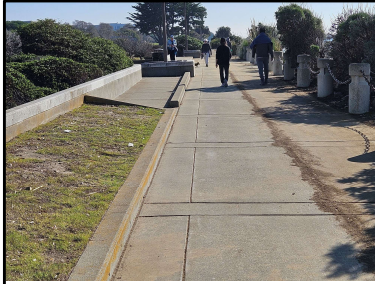
Improved trail North and South of Parcel 4
