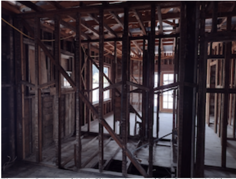
Figure 9. Interior of 1319 Clinton Avenue (GA, October 2025)
