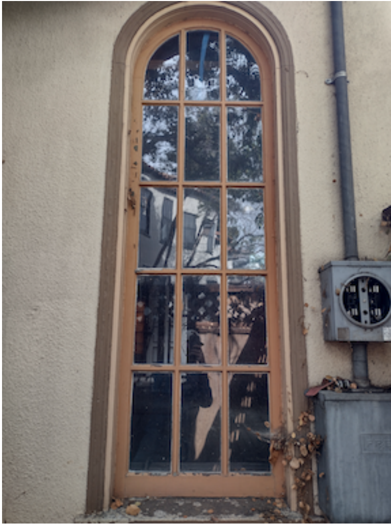
Figure 8. Arched Windows, (GA, October 2025)
