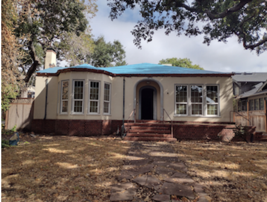
Figure 7. View of the front (South) facade of 1319 Clinton Avenue (GA, October 2025)
