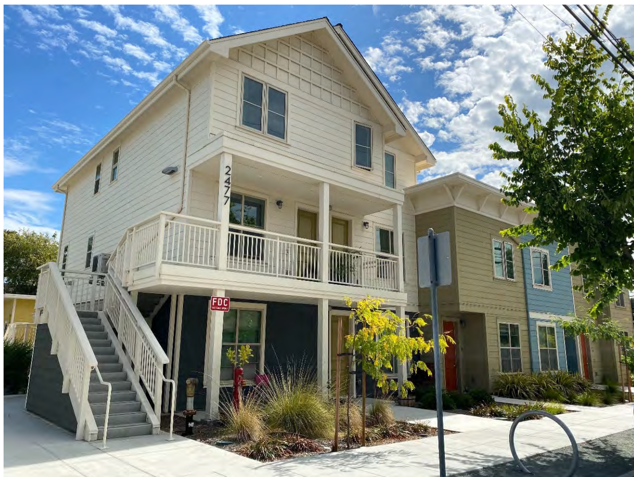
Figure 2 In 2018, the Alameda Housing Authority opened 20 units for lower income families on Eagle Avenue. The land for the project was provided by the Alameda Unified School District and the City of Alameda.
