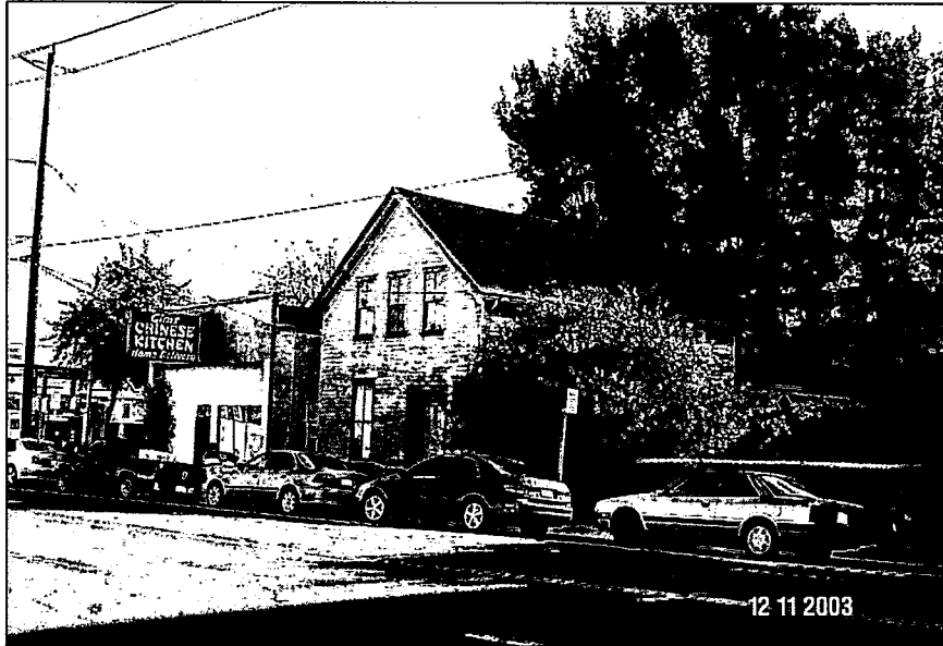
Figure 1: View Southeast of 2320 (on right) and 2322 (on left) Lincoln Avenue
