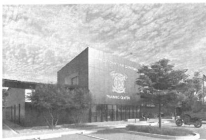
Alameda County Fire Training Center
