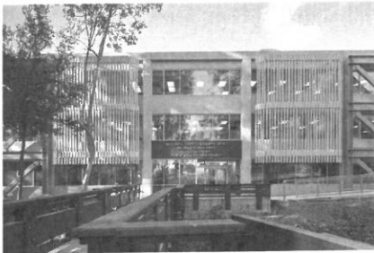
Peralta Oaks Seismic and Tenant Improvements
