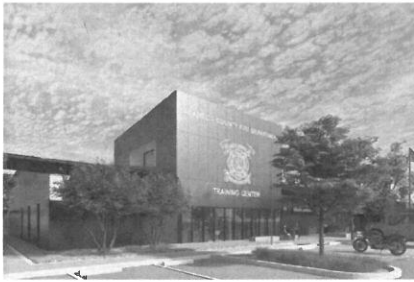
Alameda County Fire Training Center
