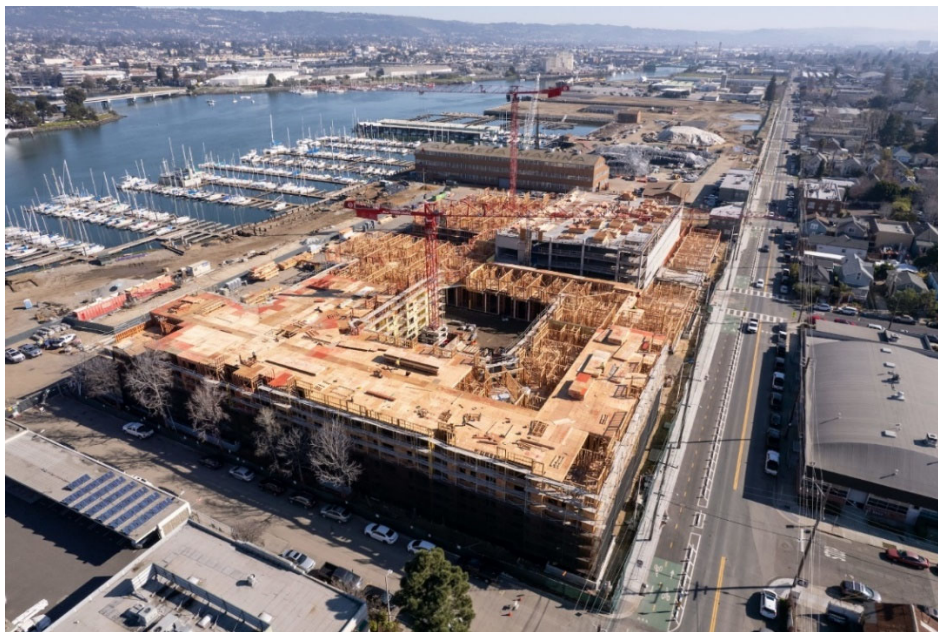
New multifamily rental housing coming online in 2022 at the Alameda Marina project on Clement Avenue.
