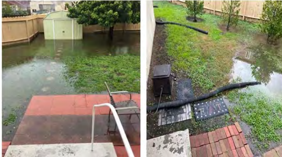
Figure 5 – December 2021 Property Flooding at 3 Garden Road
