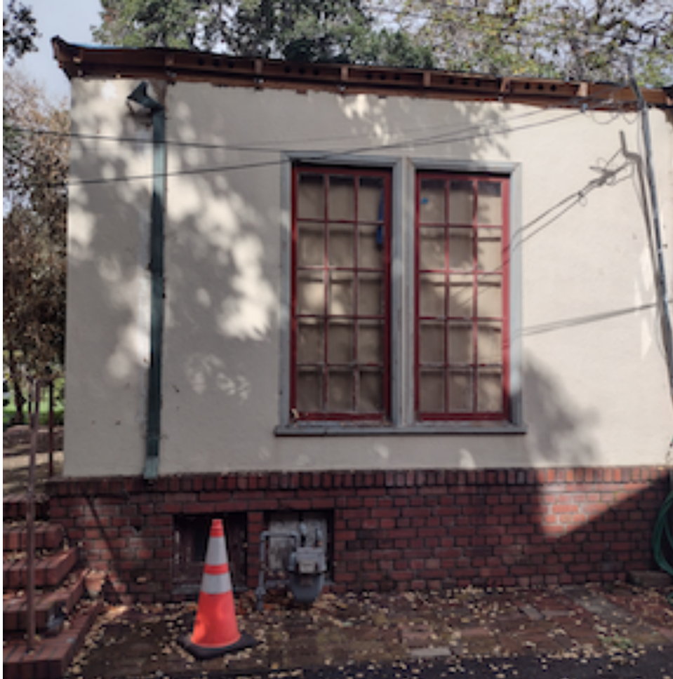
Figure 6. Wood windows on East elevation (GA, October 2025)
