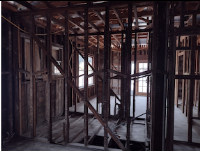
Figure 9. Interior of 1319 Clinton Avenue (GA, October 2025)
