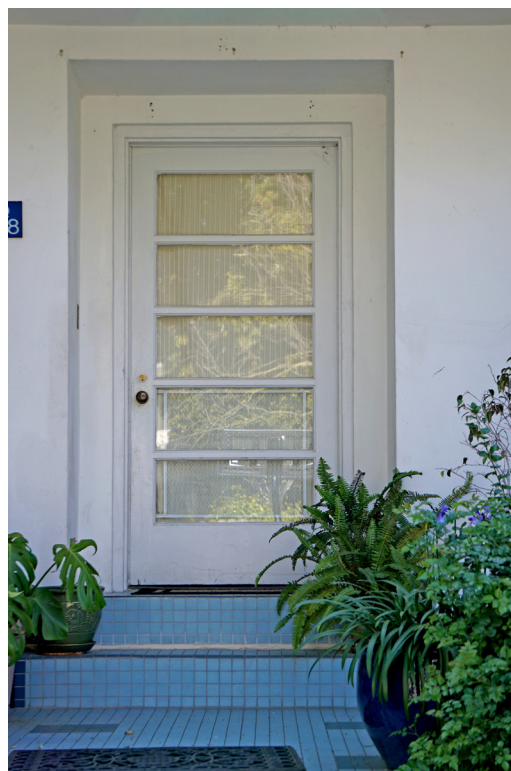
Utilize door designs that draw from configurations found elsewhere in the neighborhood
