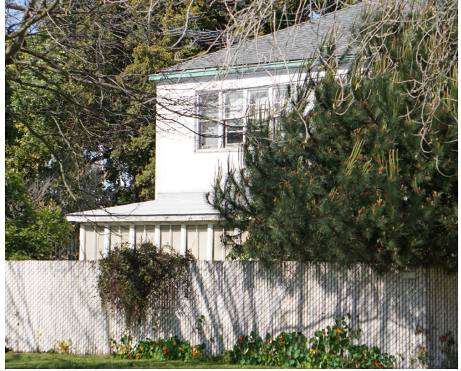
Non-historic fences are recommended to be removed in the Historic District
