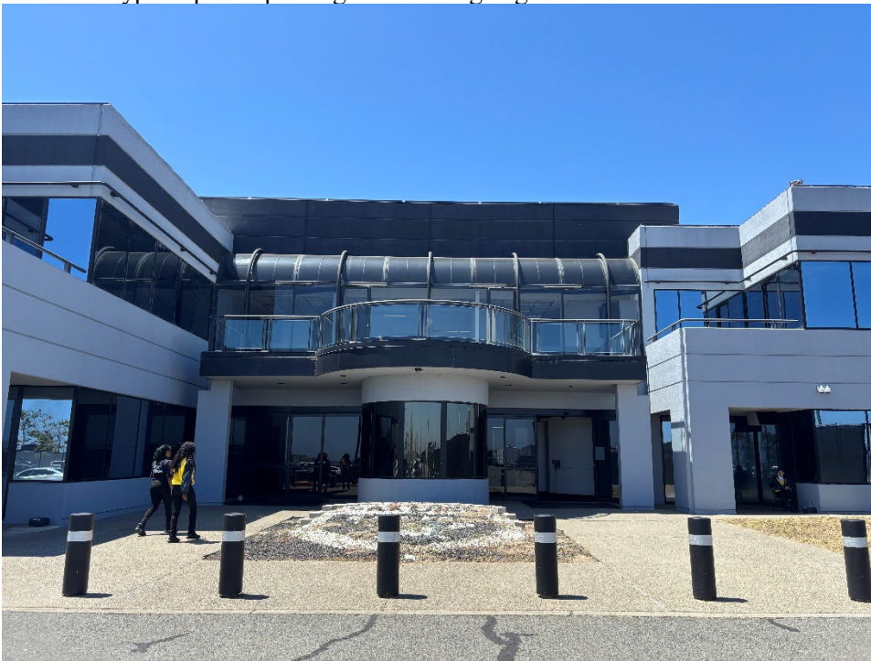
Photo 5: Modern buildings on the Project Site provide limited habitat value for wildlife..
