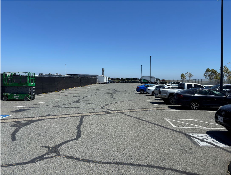
Photo 4: Typical paved parking area lacking vegetation.
