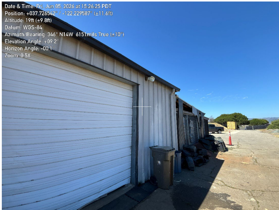
Photo 3: A house finch nest located on a speaker above and to the right of the roll-up door at the northern utility structure.
