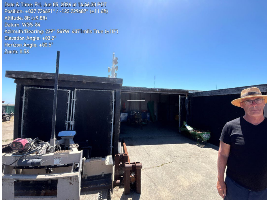
Photo 2: Swallow nests are located inside the northern utility structure, behind the open doorway shown.
