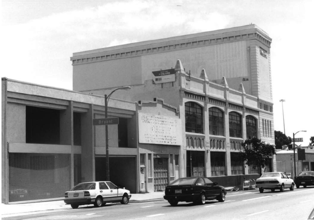
Appendix Item B. Ca. 1996 view of the Rothchild Building without addition; view toward south Source: National Register nomination by Anne Bloomfield
