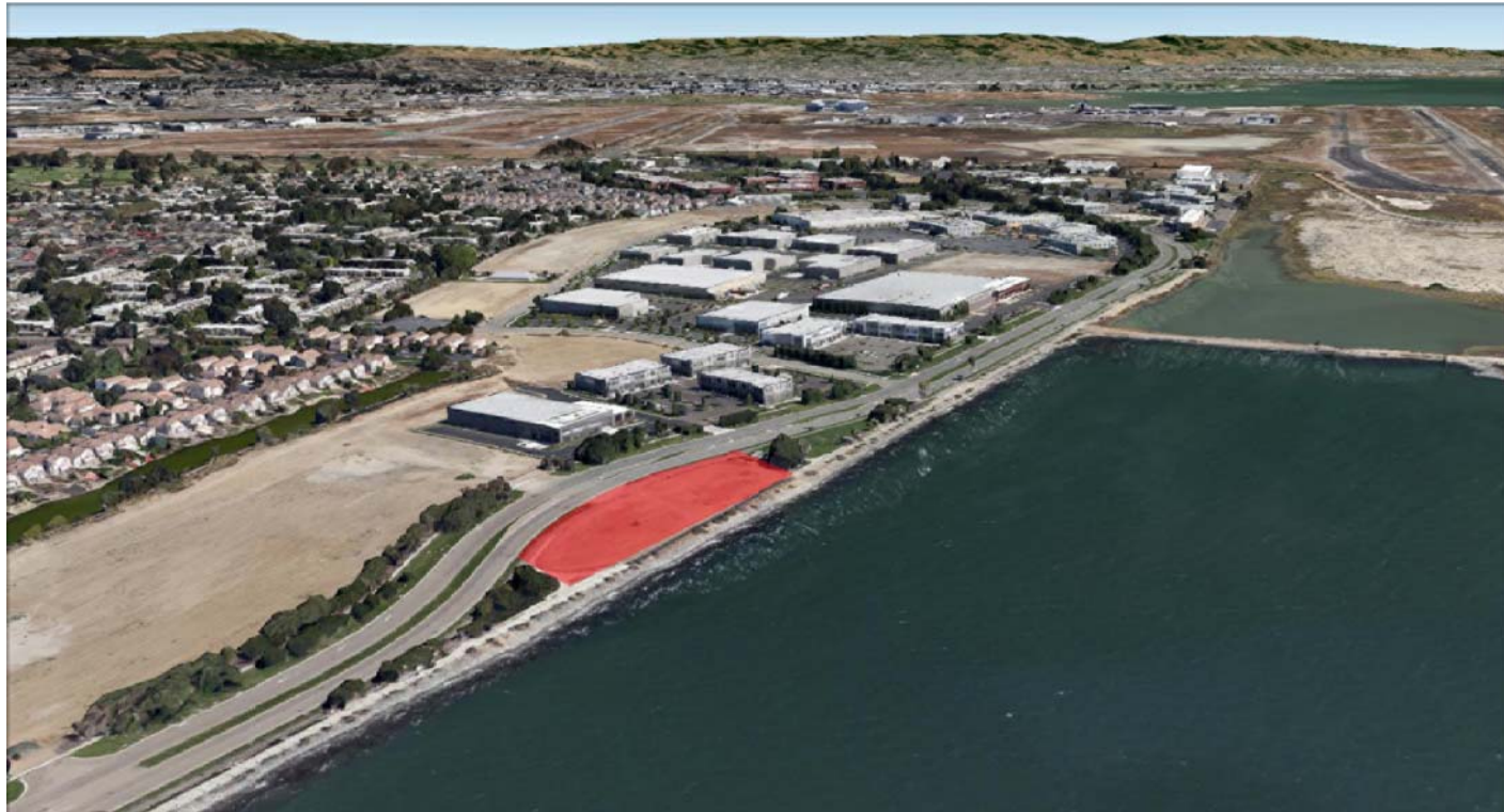
AERIAL VIEW- NORTH EAST
