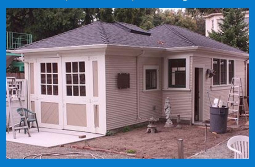
In addition to raising \$40,000 to paint the family home, the museum raised more than \$20,000 to preserve the building that the Meyers family used as a carriage house. The structure originally sat on a mud sill, and 110 years of weathering, dry rot and termites had brought the building to the point of collapse. Today, rebuilt walls rest more permanently on a concrete slab. The museum plans to use the renovated space to display items from its collection.
