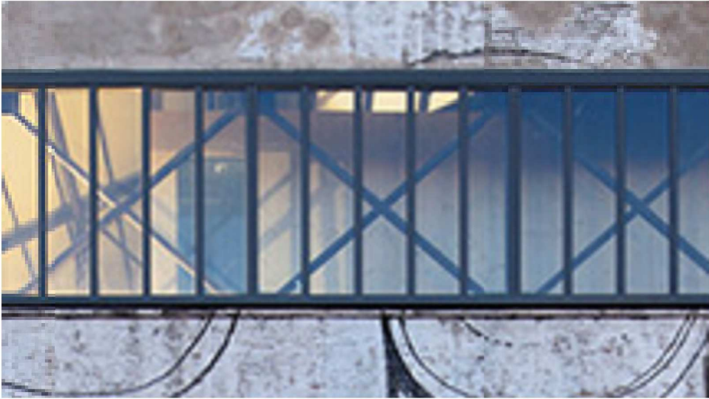
NEW RIBBON WINDOWS AT 2ND FLOOR, BUILDING 9
