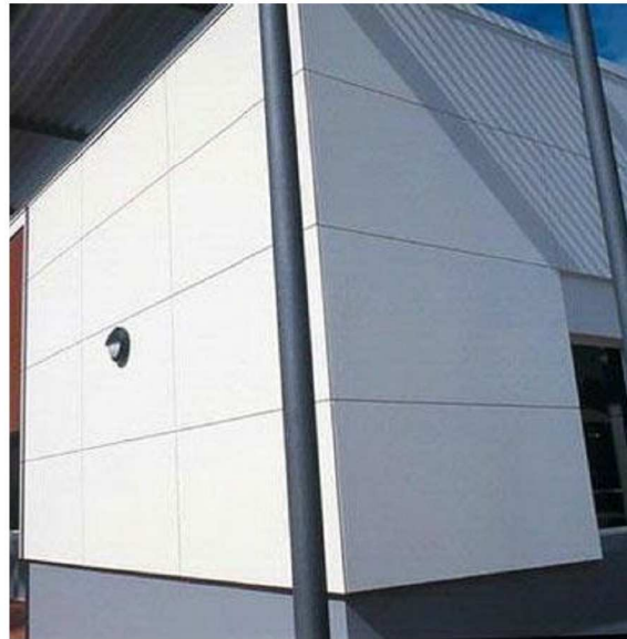
FIBER CEMENT PANEL WITH CONTRASTING BASE AT BUILDING 91 ADDITION
