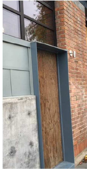
EXTENDED FRAME AT NEW ENTRY, BUILDING 9
