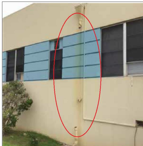
City Hall West – Missing downspout
