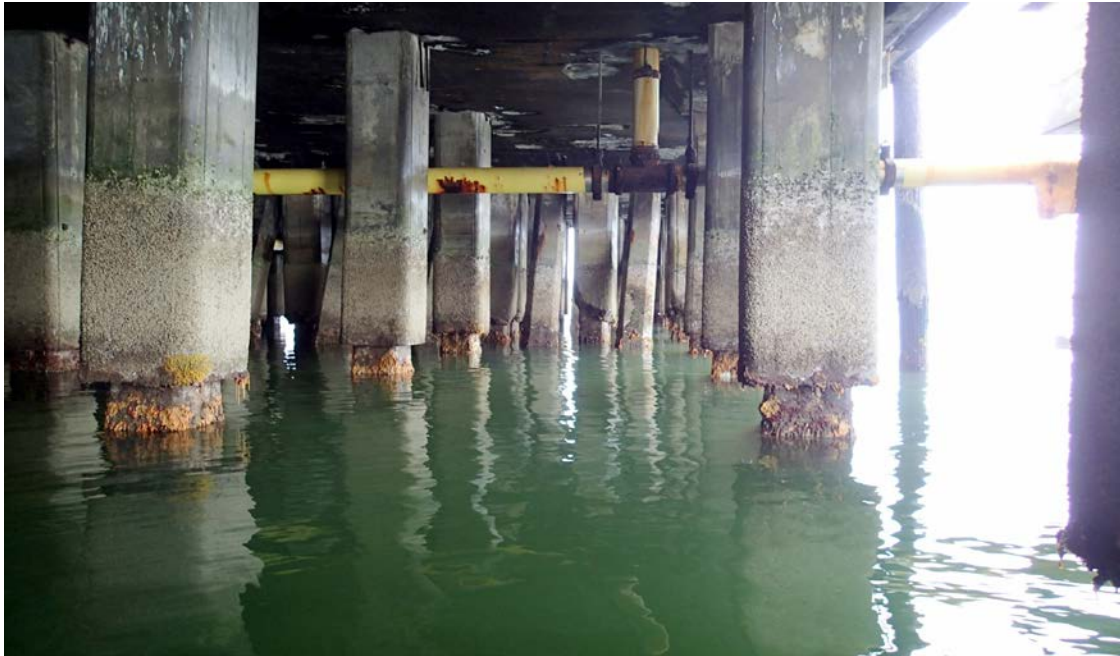
Typical Piles Bents_offshore
