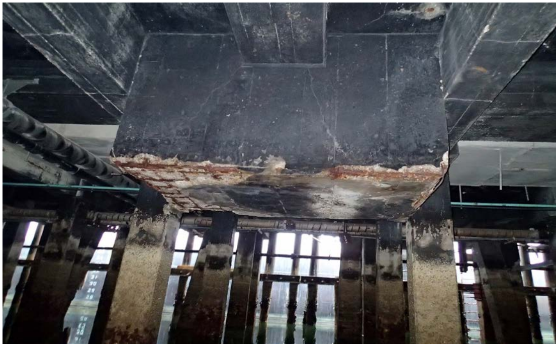
Spall and Rebar_Utility Vault
