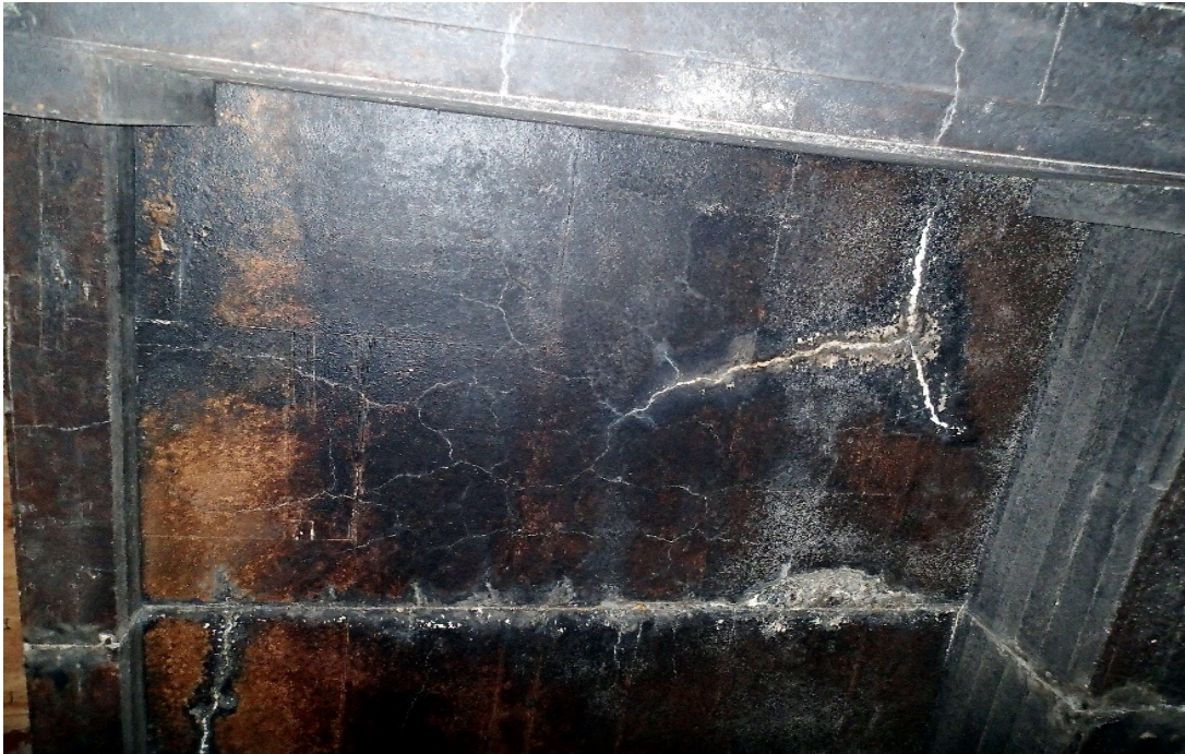
Underdeck cracks
