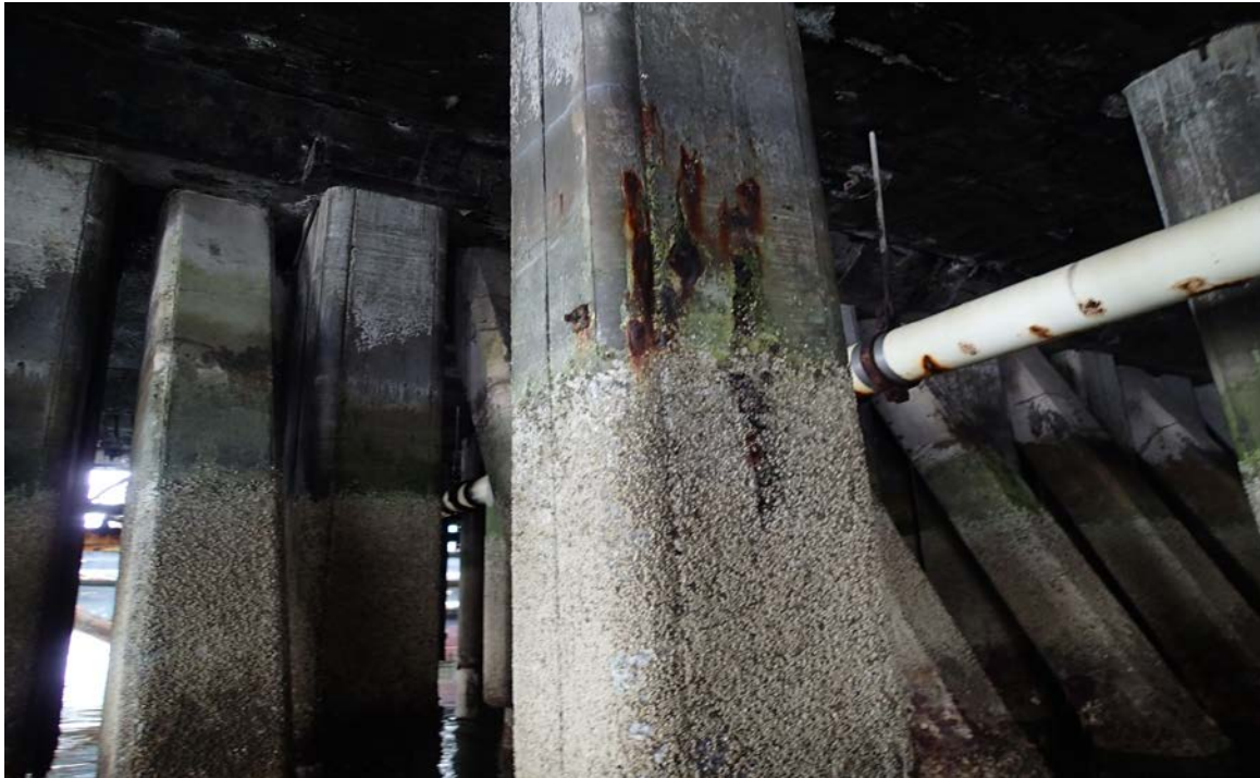
Typical Pile Corrosion Staining
