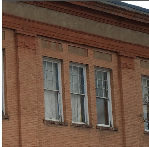
COLUMN, LINTEL & SPANDREL EXAMPLES
