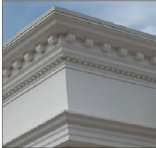
CORNICE DENTIL BLOCK EXAMPLE
