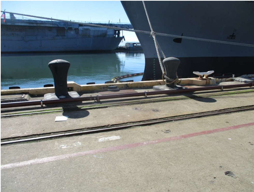
Photo 19 – New bollards at Pier 2
