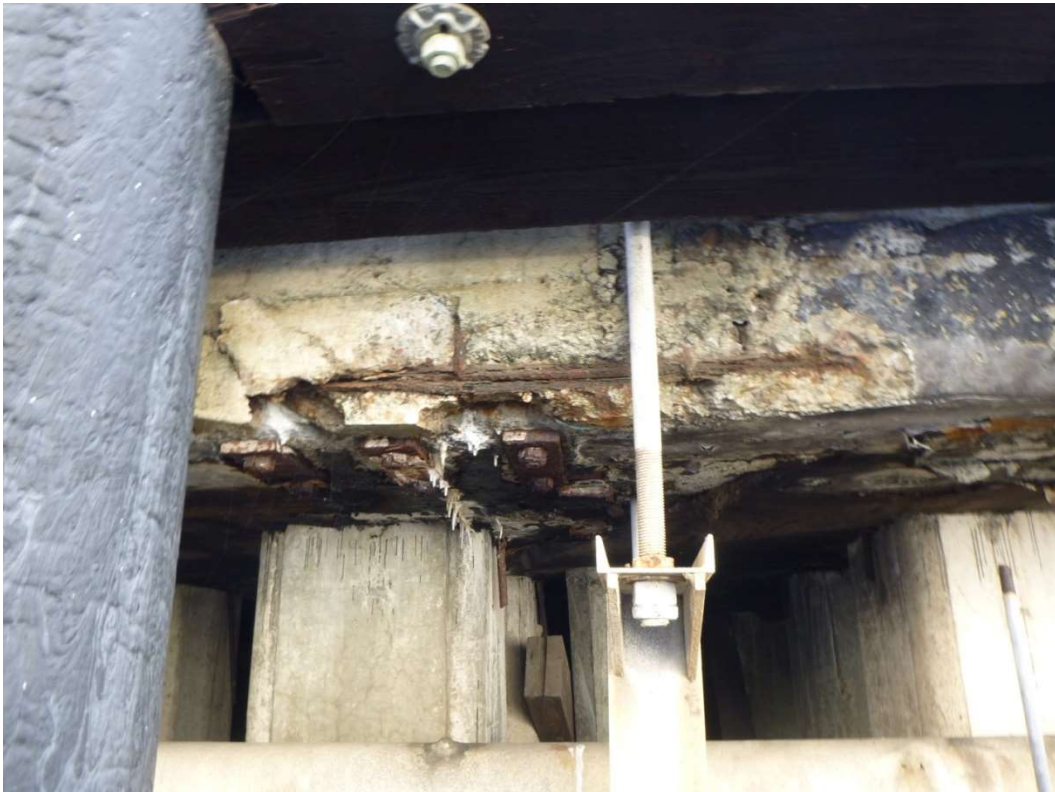
Photo 24 – Corrosion spalling of deck edge at Pier 3
