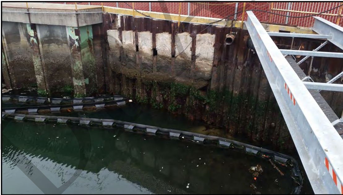
Photo 6: Original steel sheet pile wall at south side of Pier 1.
