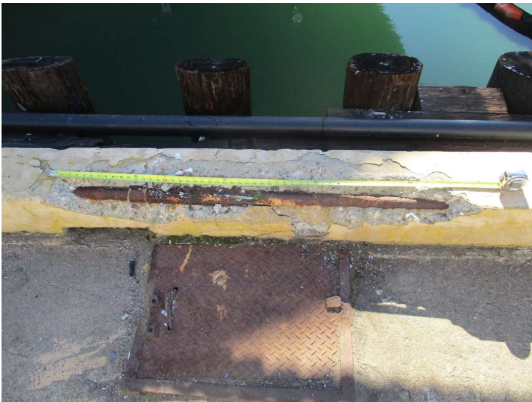
Photo 20 – Spalling of curb at Pier 2
