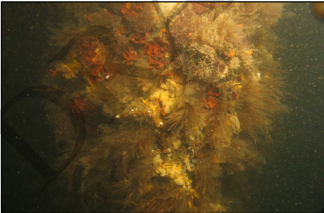
Photo 4: Typical marine growth on structural piles.
