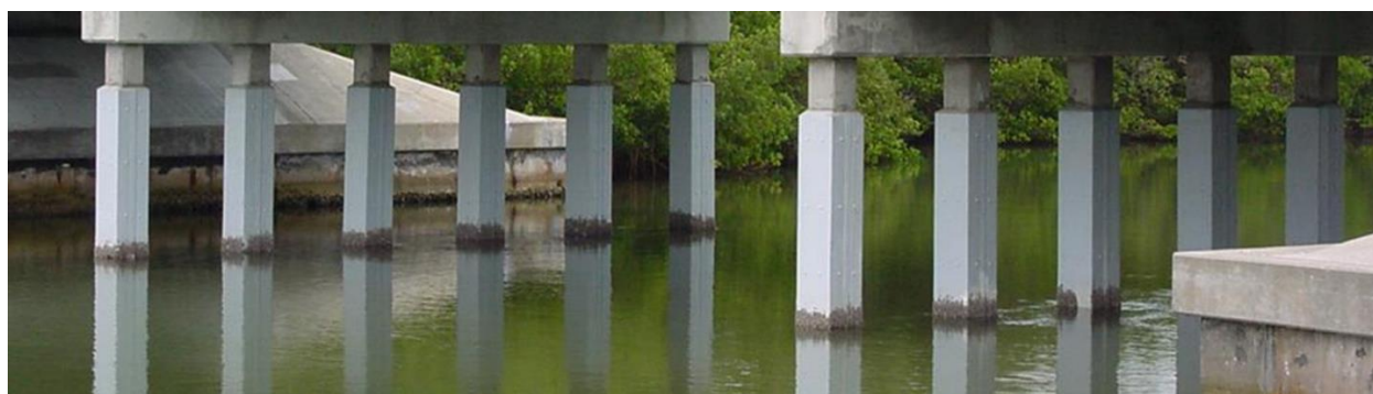
Figure 1: Pile Repair Jacket Option
