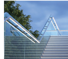
2 Handrail integrated stair lighting
