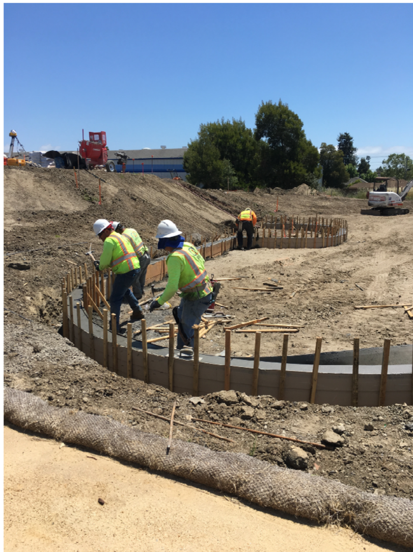
Concrete forming for curbs in playground area with sliding hill seen in the background.
