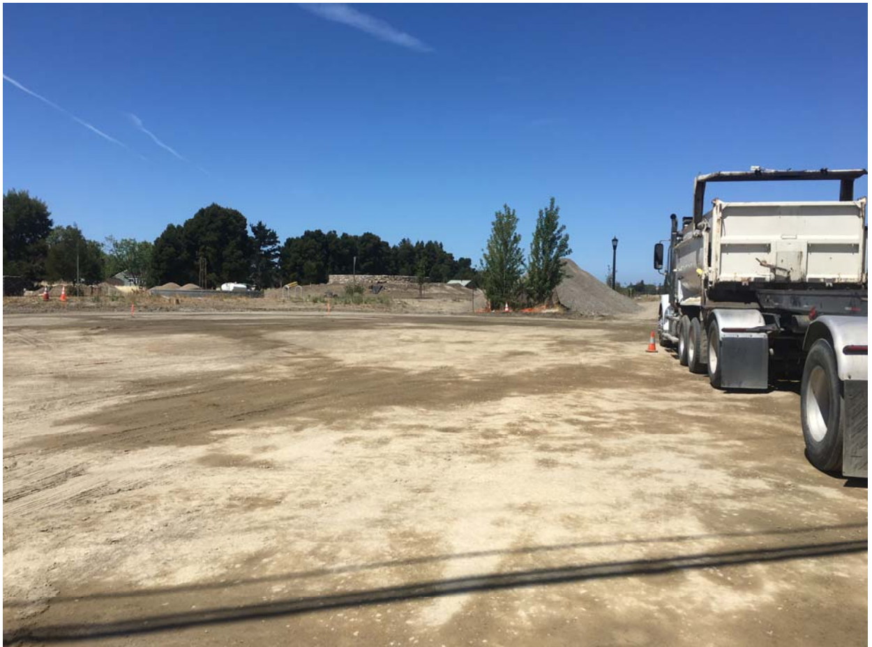
Grading complete for parking lot and ready for compaction testing.
