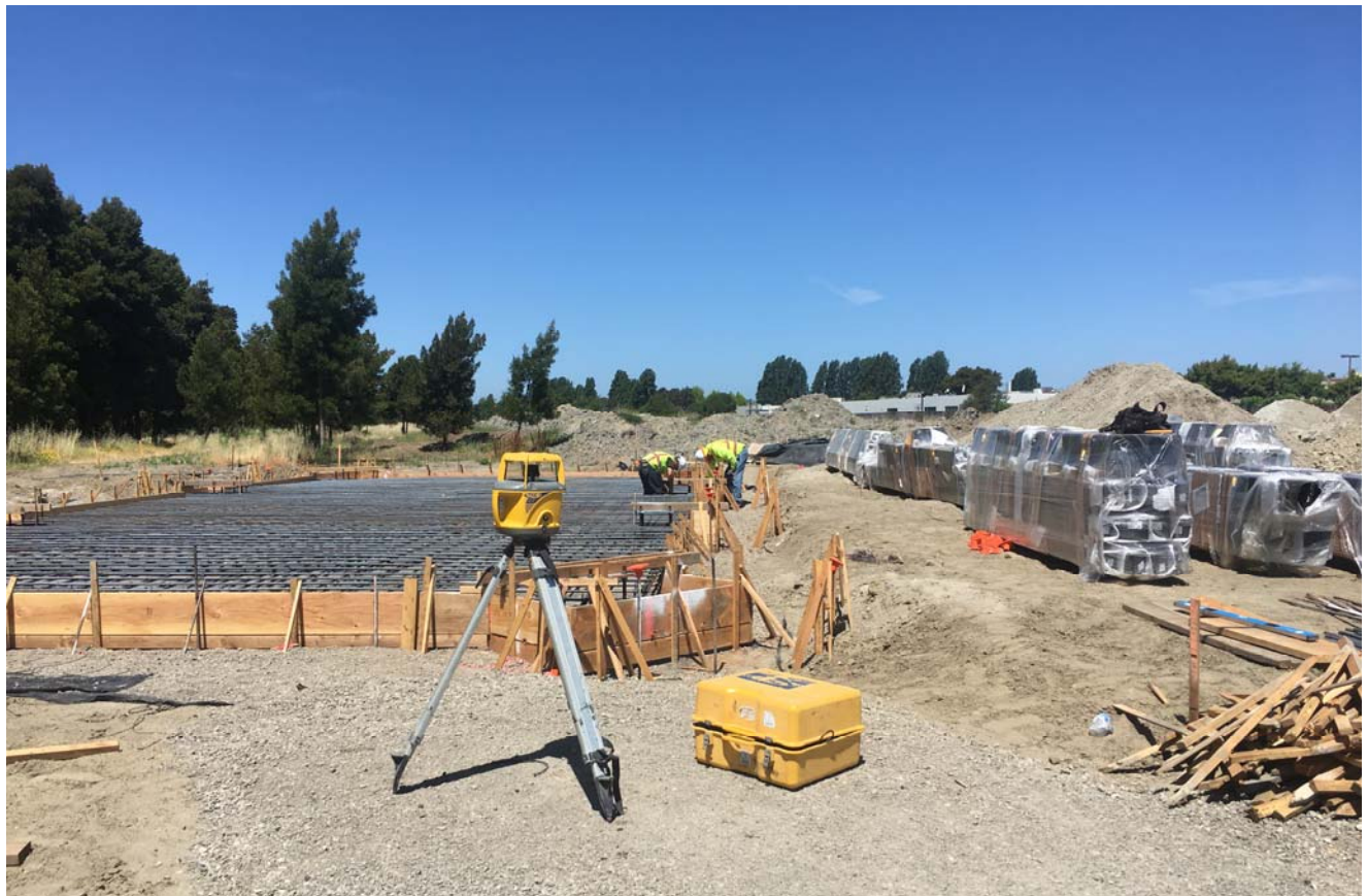
Concrete forming for Rotary Picnic Pavilion with pavilion parts on right side.
