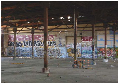
Timber framing in existing warehouse to be removed
