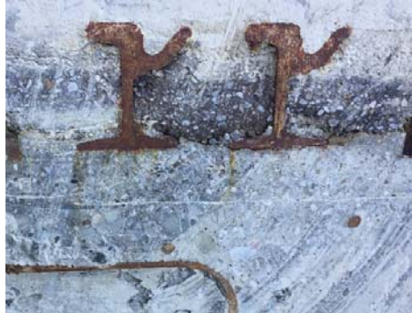
Section cut through existing girder rails
