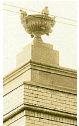
Decorative urn from roof parapet, from photo circa 1929. Urns were removed in 1956 after a portion of the parapet wall collapsed. This enhanced photograph provides enough detail to create a replica of the urns.
