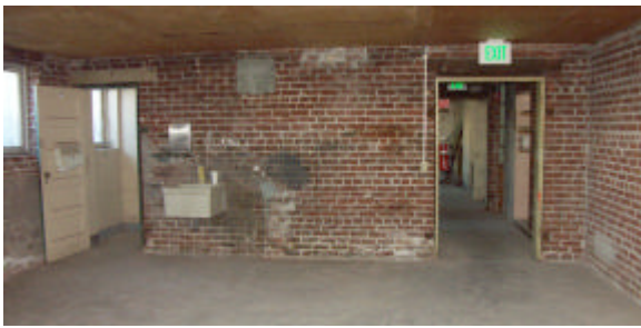
Insulation could be applied to historic exposed brick exterior walls in the basement. Interior walls would remain brick.
