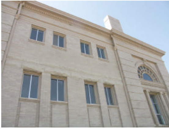
Above: aluminum windows on the East elevation.
