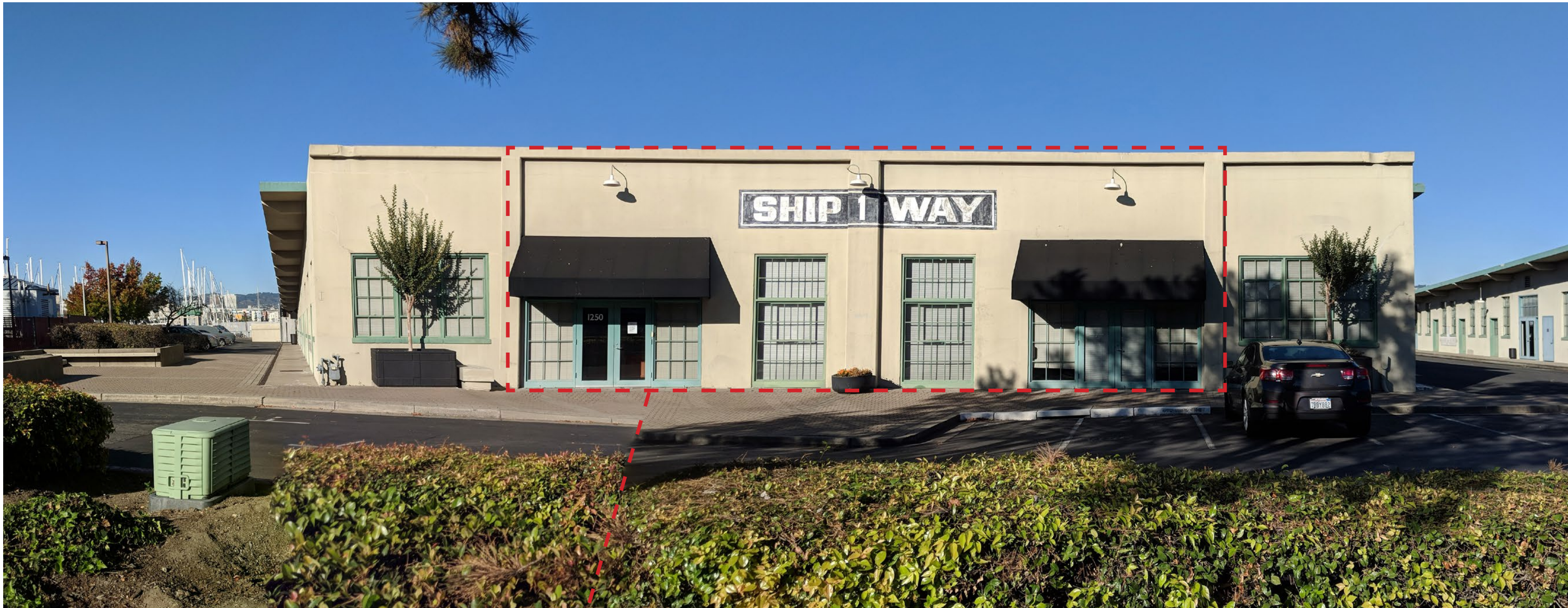
Center Facade Elements from Shipways 1 & 4 to be removed and re-installed at each corner
