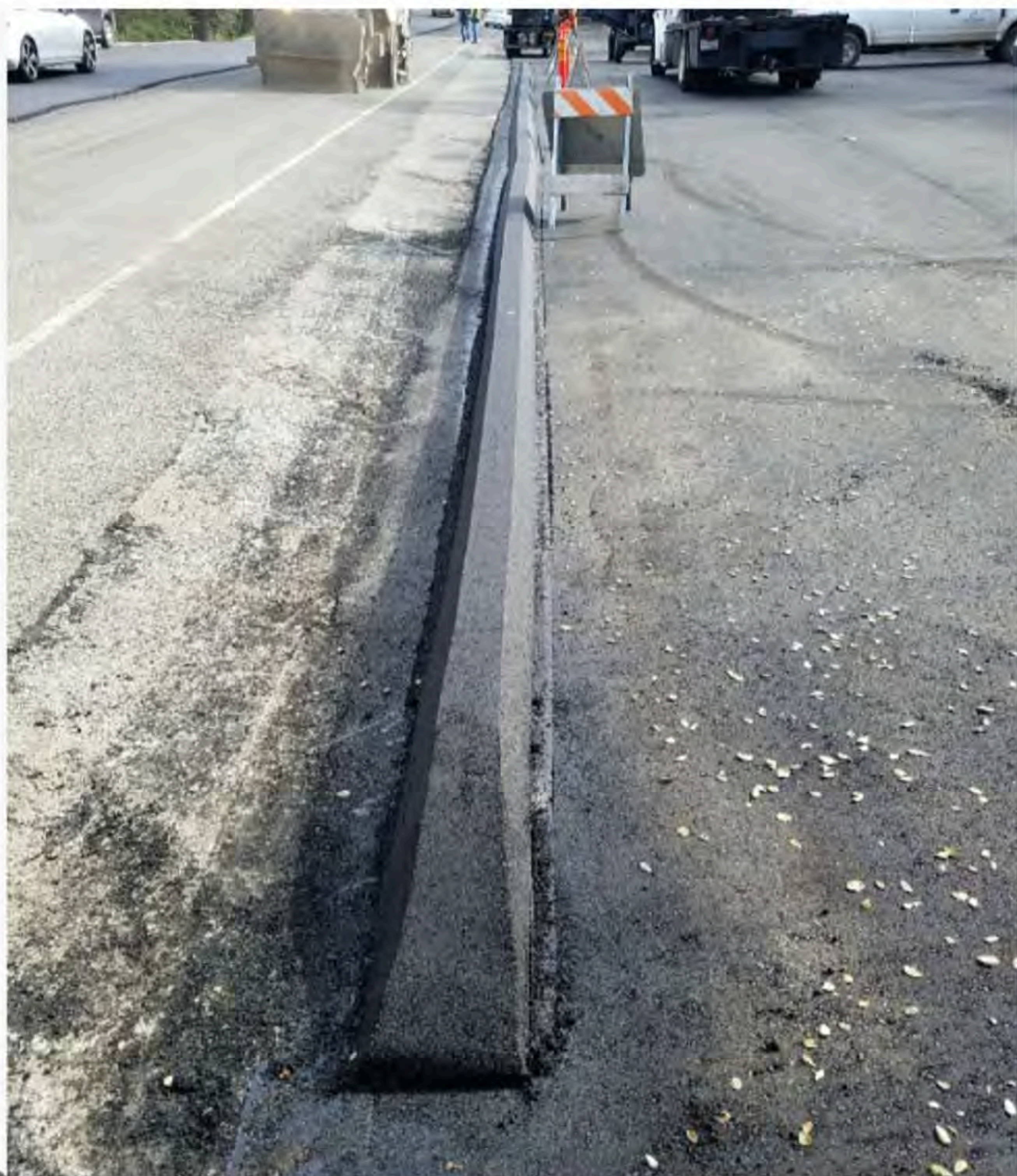
Figure 1. Temporary Asphalt Curb
