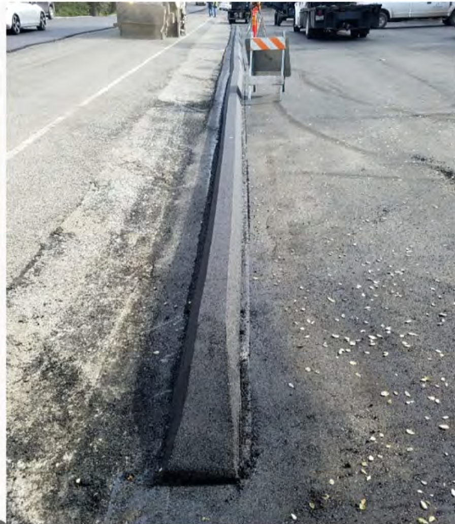
Figure 1. Temporary Asphalt Curb
