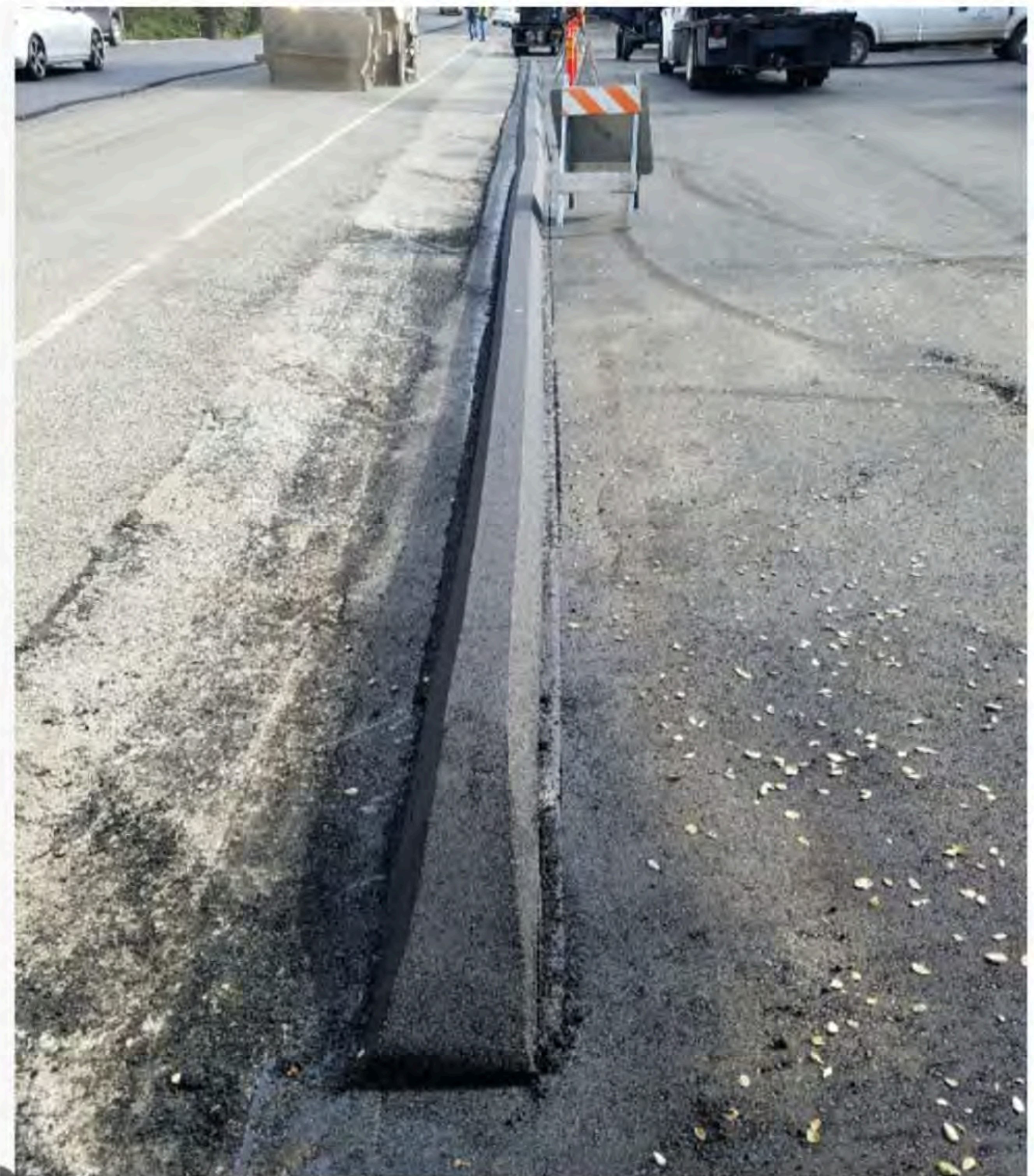
Figure 1. Temporary Asphalt Curb
