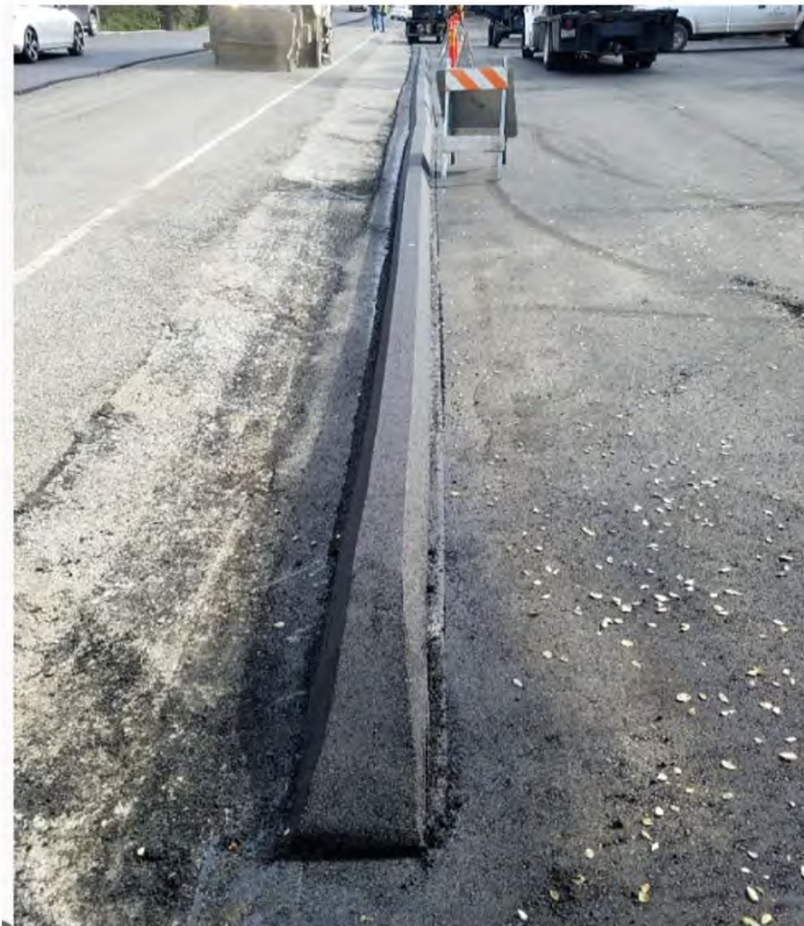
Figure 1. Temporary Asphalt Curb
