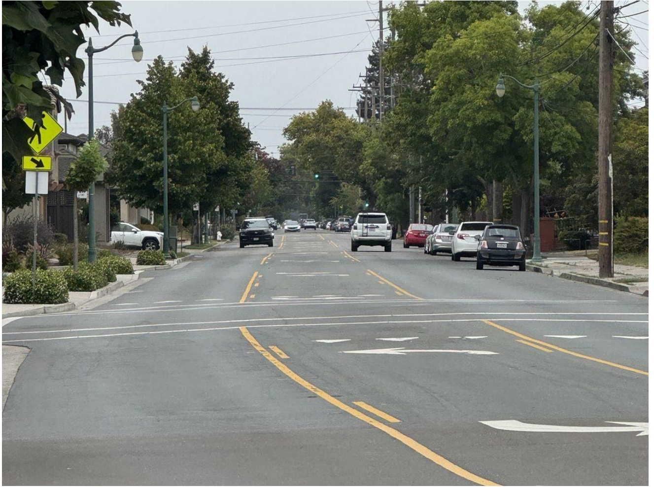
Buena Vista Avenue, the current truck route — a straight shot with no curves, ending at a signal.
