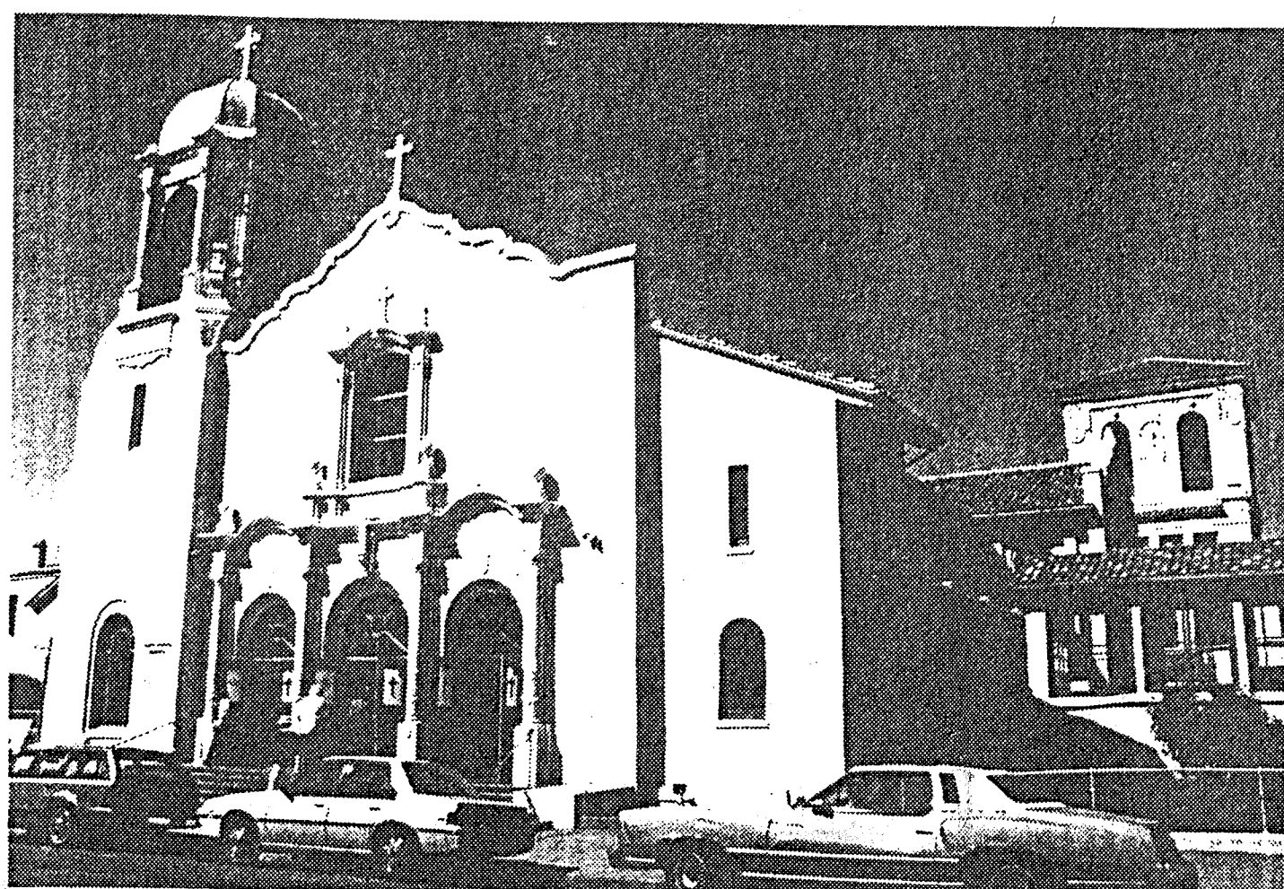
East and North Facade w/Parish Hall Entry in foreground and High School Bell Tower in background, 1989
