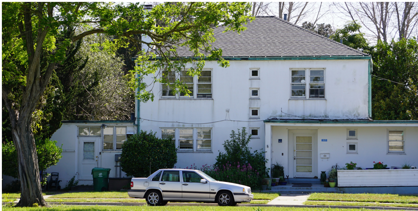
The traditional patterns of window and door openings should remain important influences when new buildings are designed
