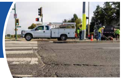
Repairing Alameda streets making them safer for pedestrians, drivers, and cyclists
