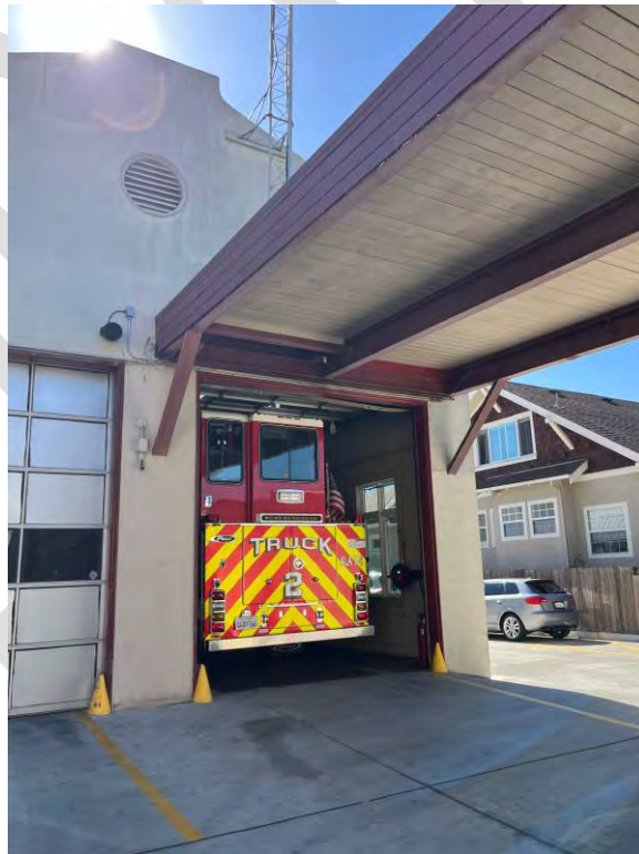
Photo 6: Steel Canopy at App Bay Wall
