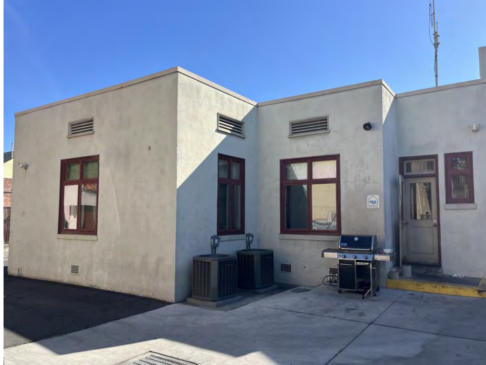
Photo 3: Fire Station North Face at Office/Residential
