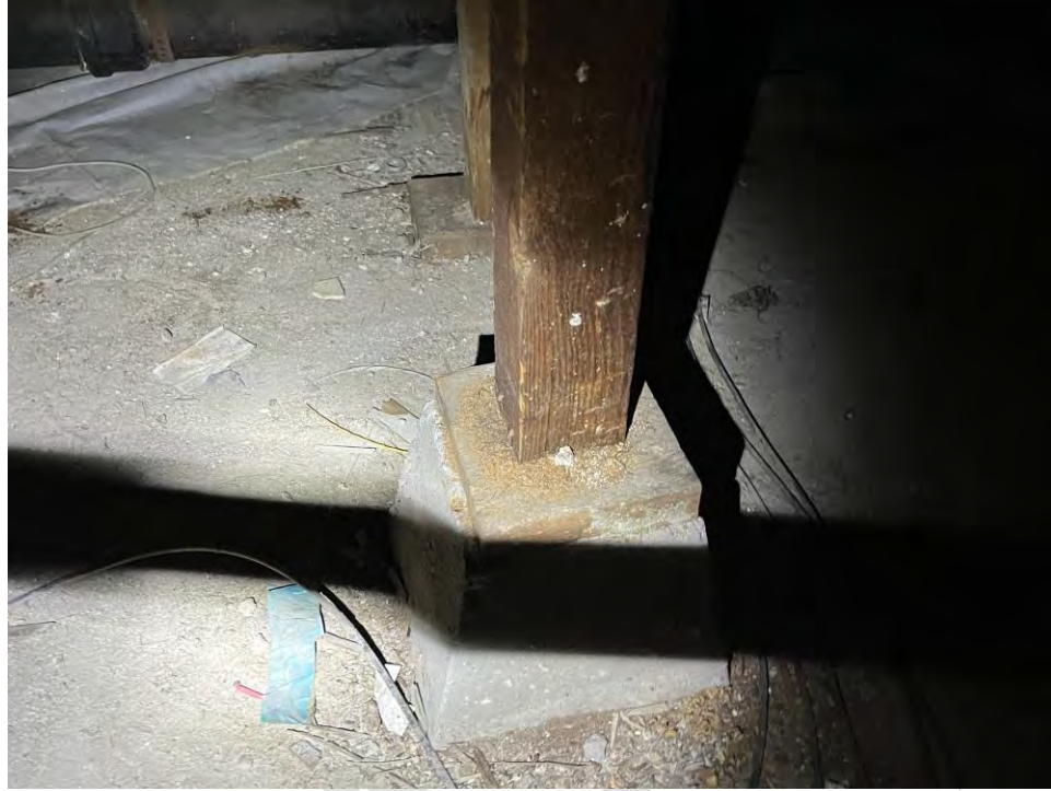
Photo 17: Column and Isolated Footing at Crawl Space
