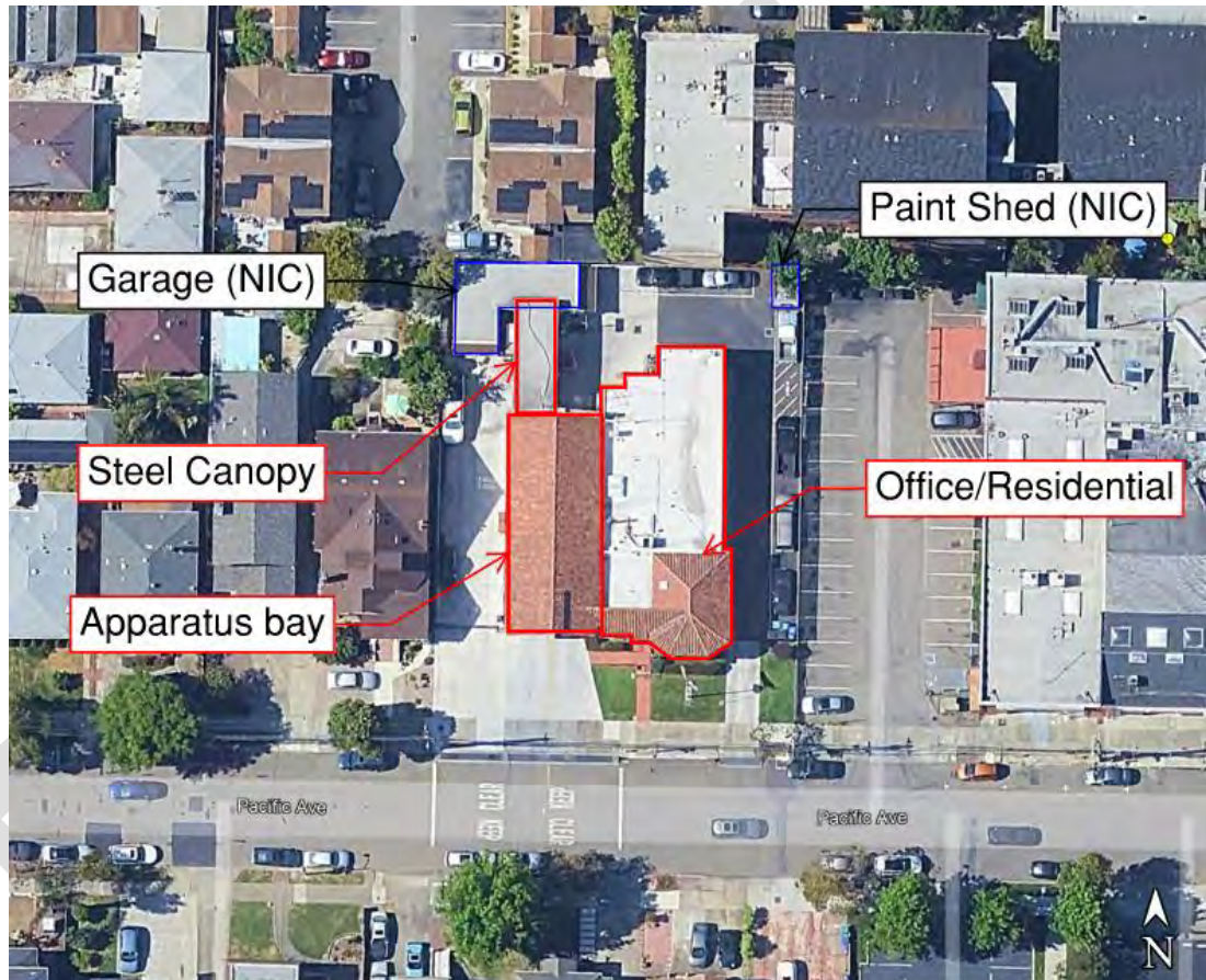
Figure 1: Aerial View of the Alameda Fire Station No. 2
