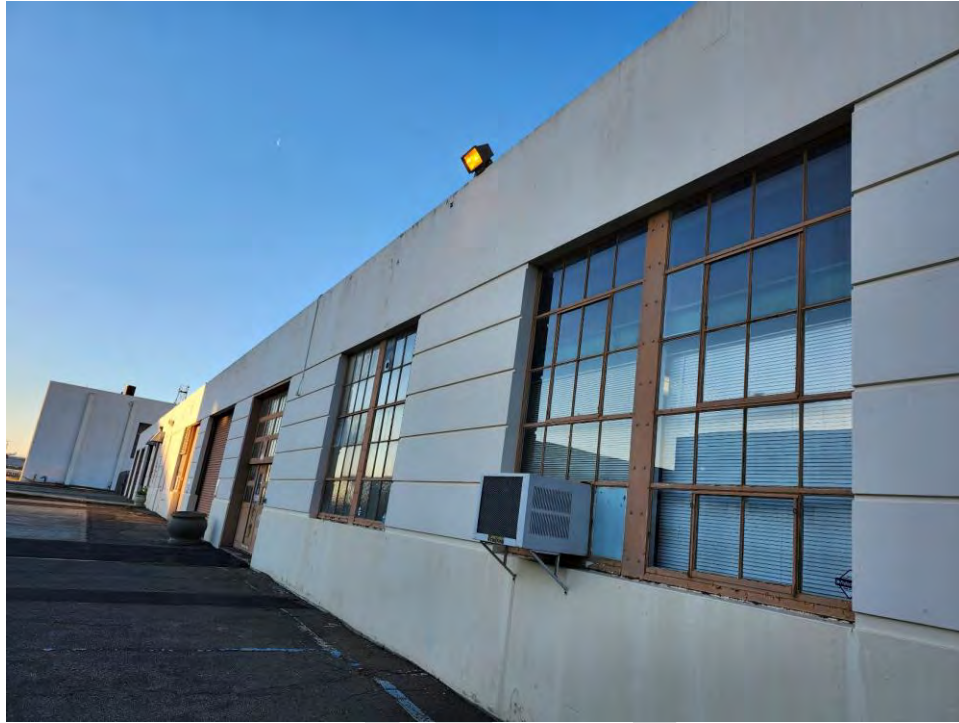
Photo 3: Eastern Face of Building
