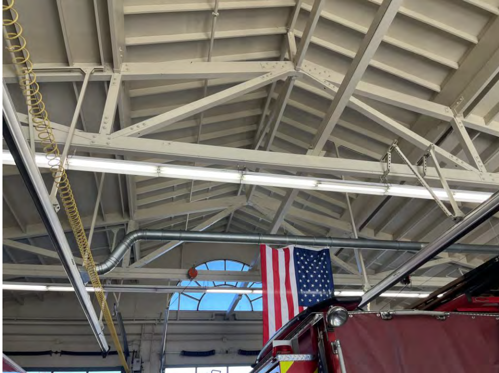
Photo 3: Apparatus Bay Roof Framing
