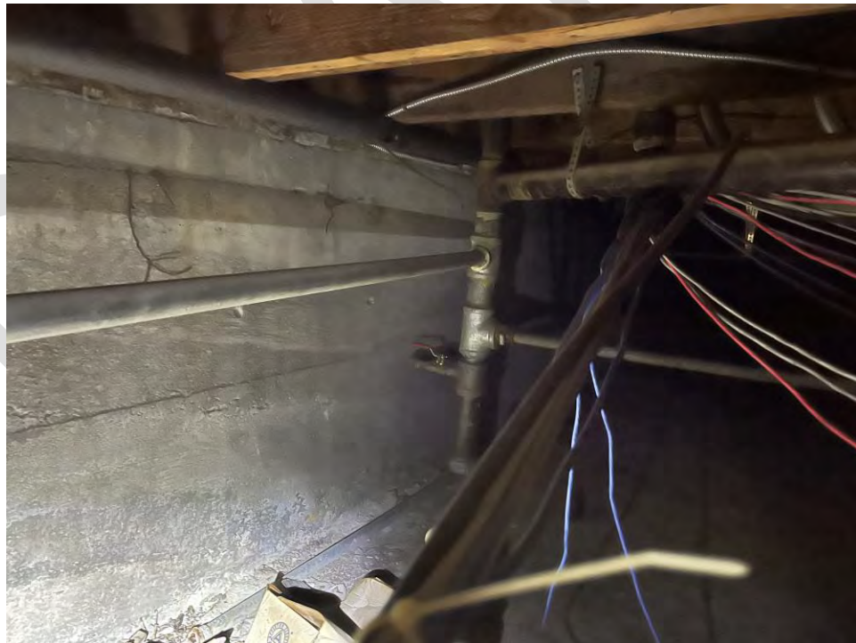
Photo 16: Floor Joists at Concrete Foundation Wall at Crawl Space
