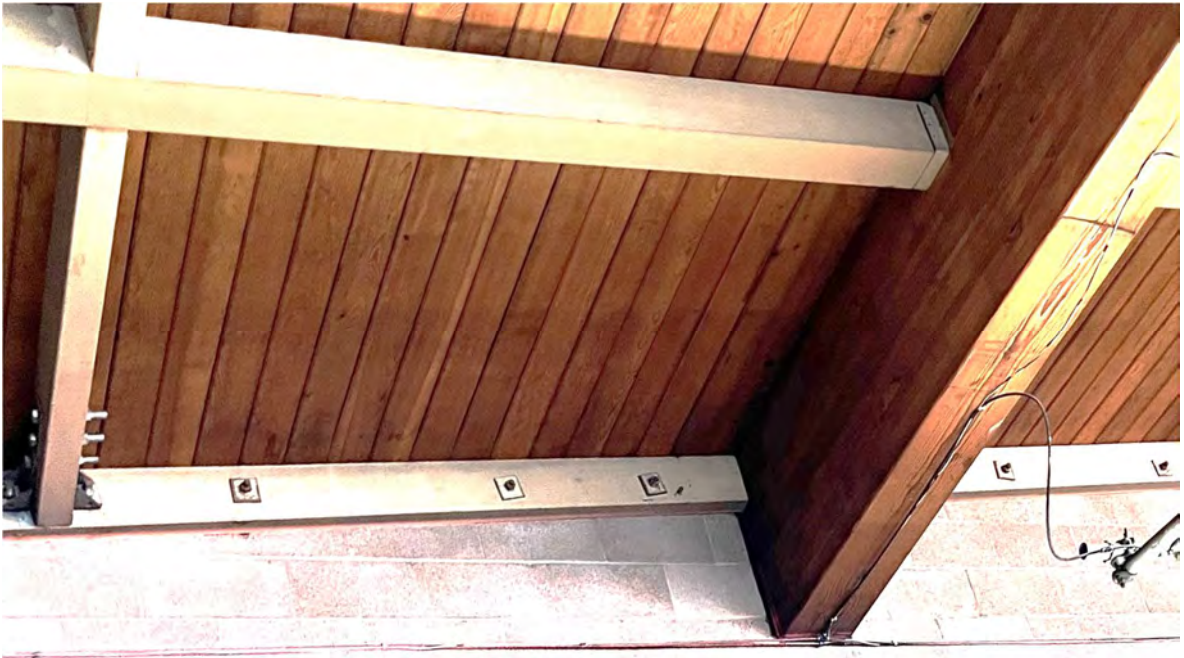
Photo 5: Apparatus Bay – Glulam to Wall Connection
