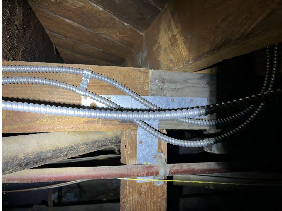
Photo 15: Joists at Beam and Column at Crawl Space
