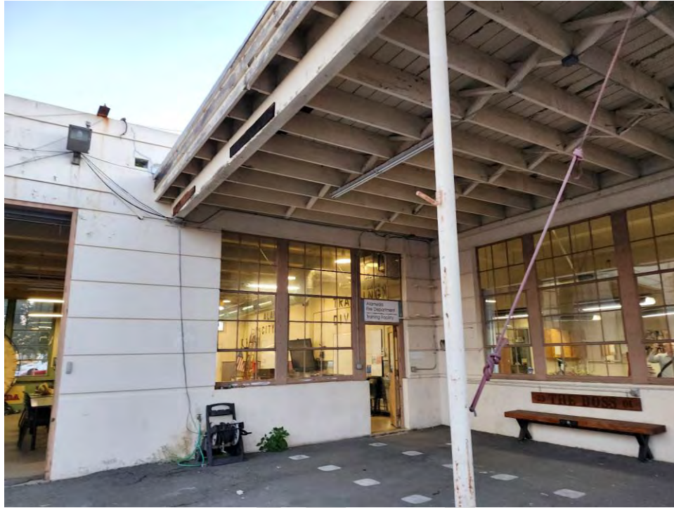
Photo 5: Wood Shade Structure
