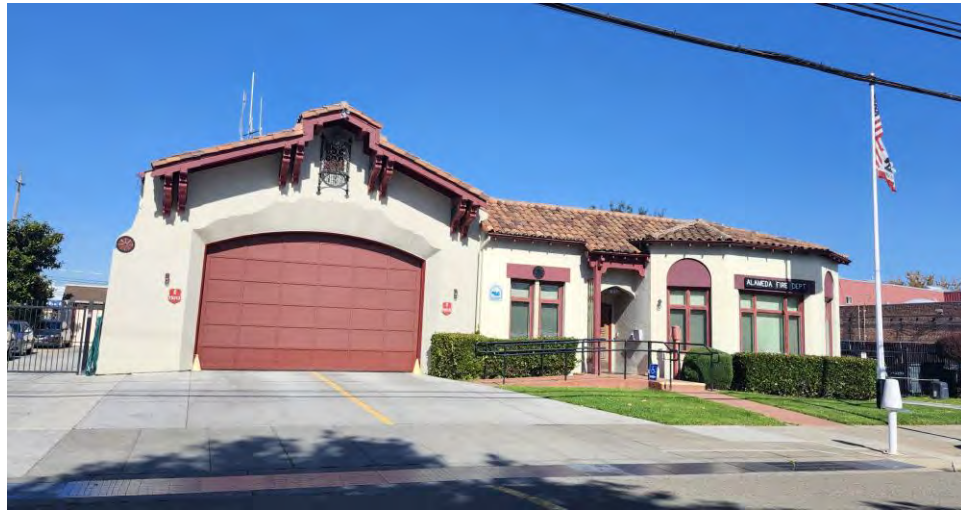
Photo 1: Fire Station South Face
