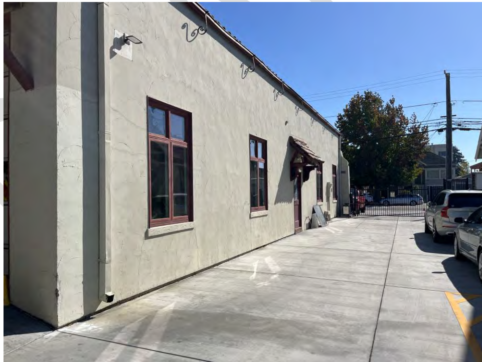
Photo 4: Fire Station East Face
