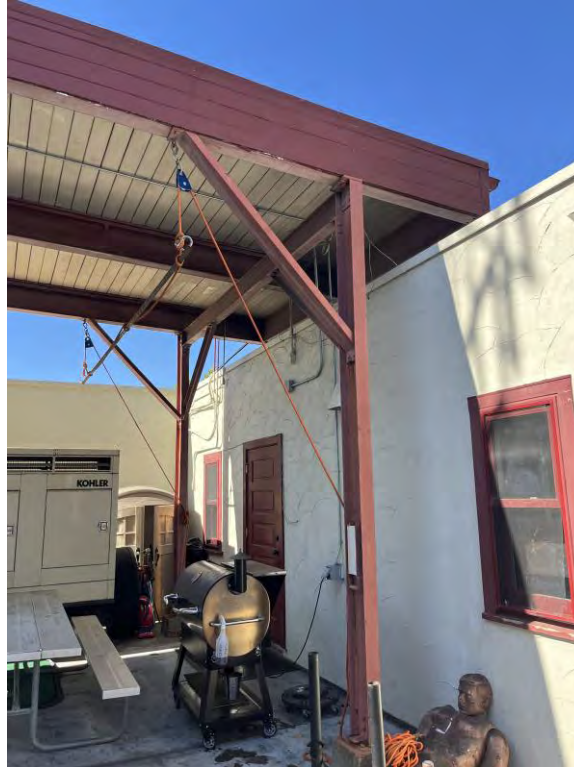
Photo 7: Steel Canopy at Garage
