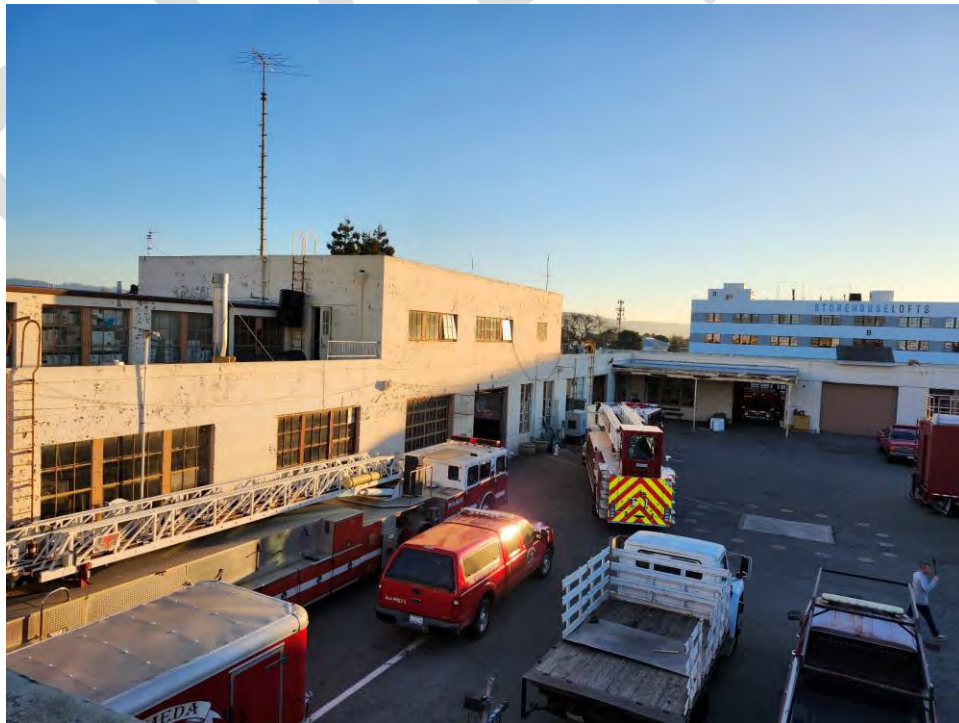
Photo 2: Southern Face of Building
