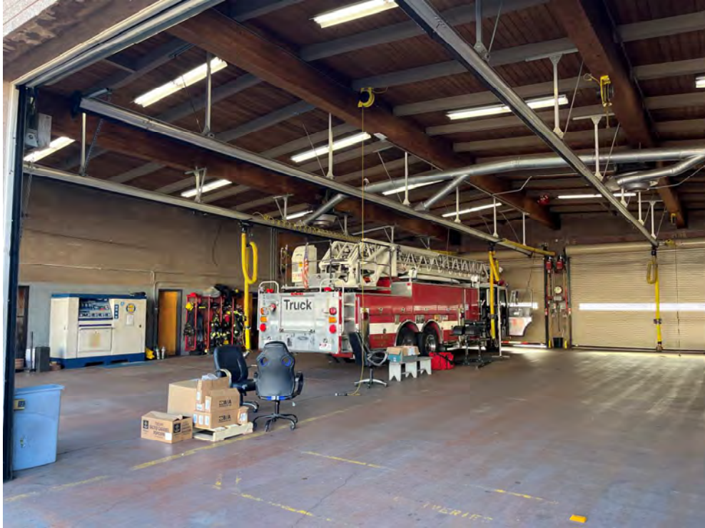
Photo 3: Apparatus Bay Roof Framing
