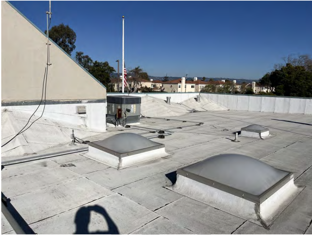
Photo 7: Roof of Main building
