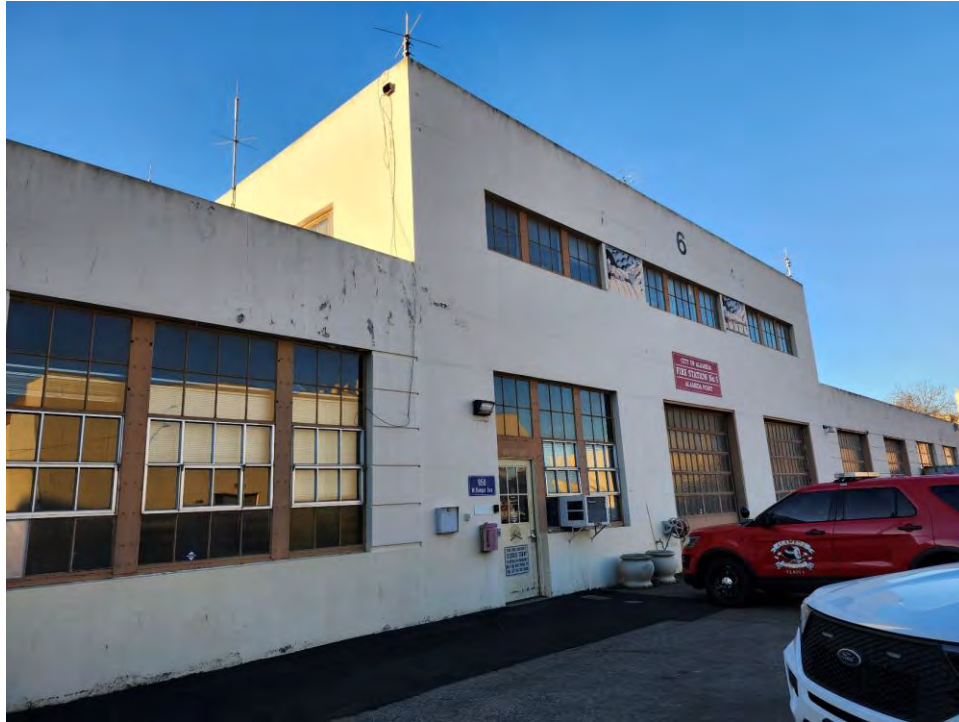
Photo 1: Entrance to Building on Northern Face
