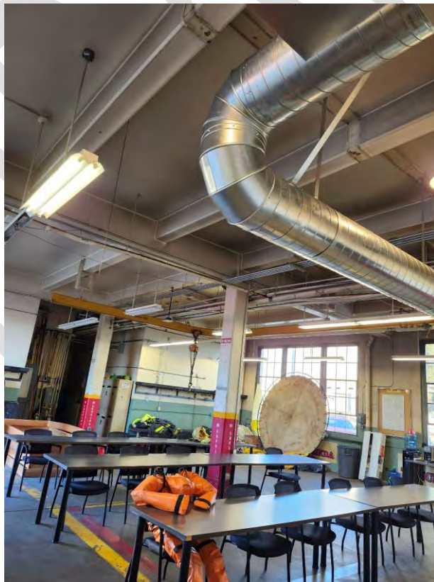
Photo 6: Concrete Roof/Ceiling Framing at Classroom
