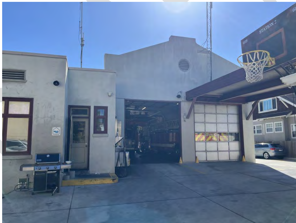
Photo 2: Fire Station North Face at App Bay
