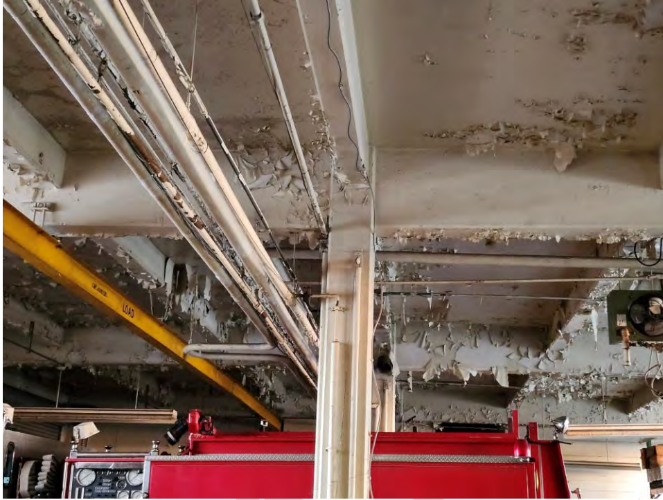
Photo 7: Concrete Roof/Ceiling Framing at Storage Apparatus Bays
