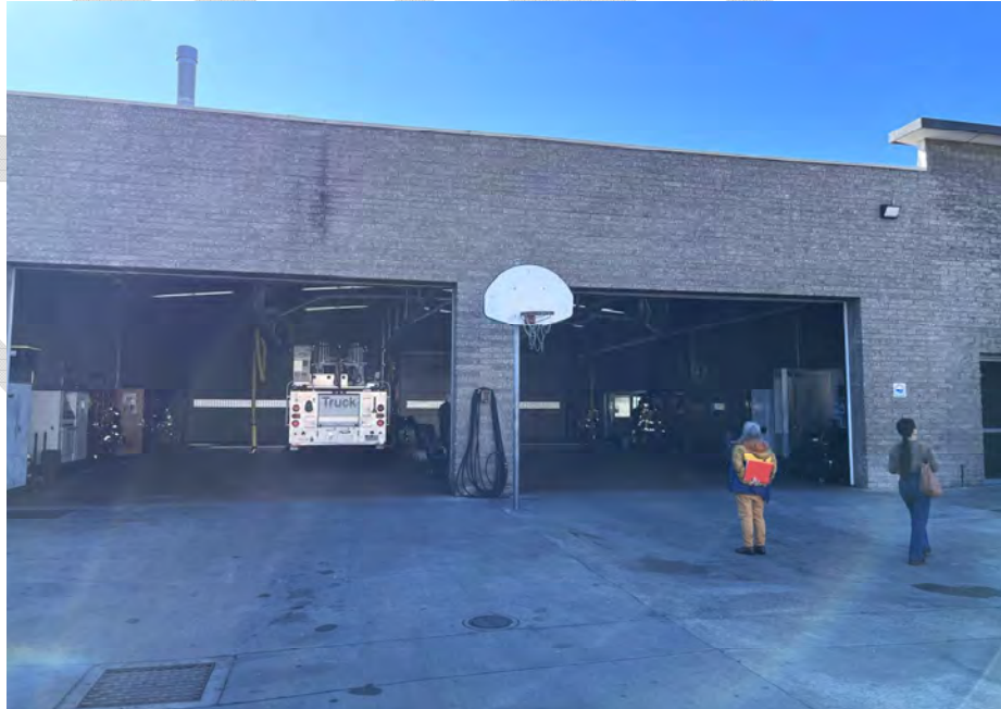
Photo 2: Apparatus Bay Entrance
