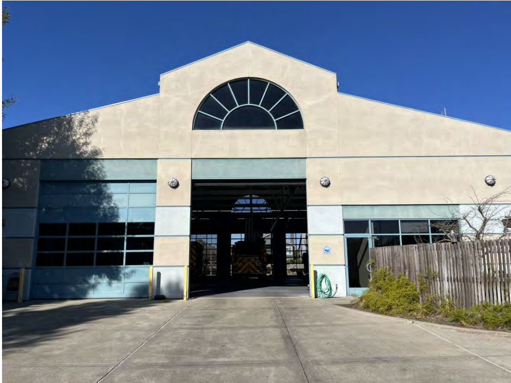
Photo 1: Apparatus Bay Entrance
