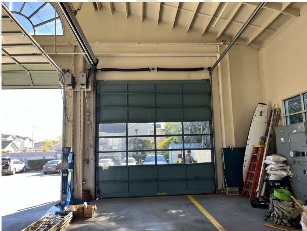
Photo 4: Apparatus Bay – Steel Moment Frame
