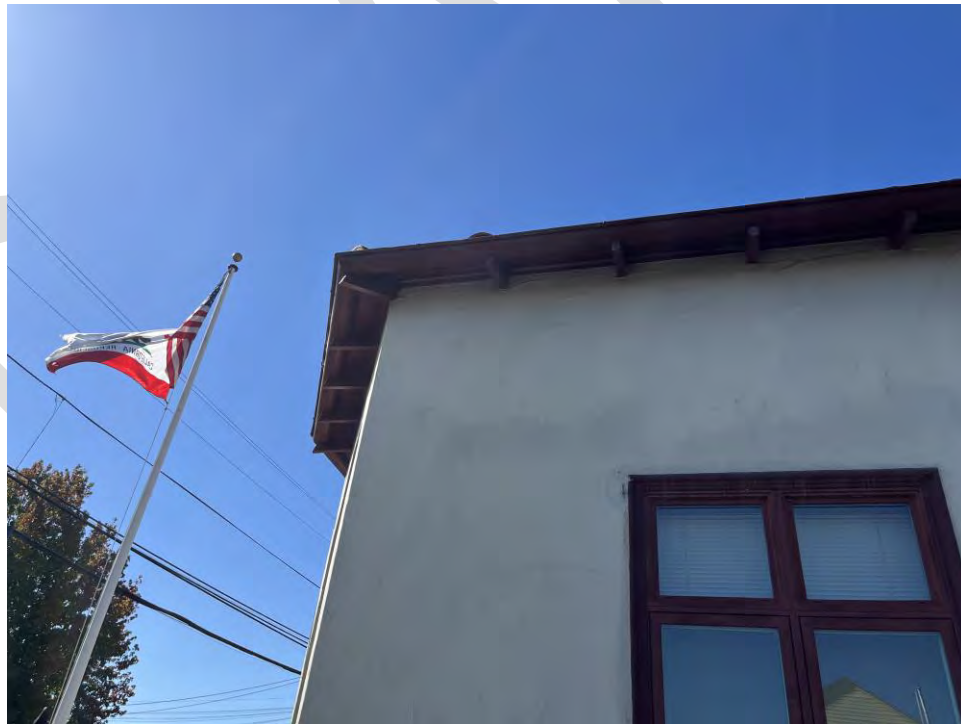
Photo 12: Exterior Soffit at Clay Tile Roof Overhang
