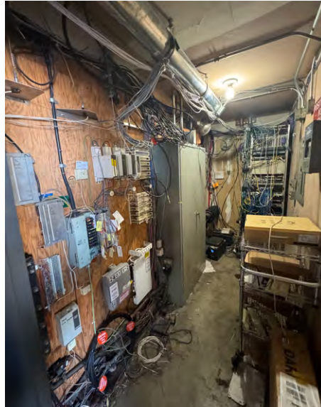
IMAGE C - EXISTING TELECOM ROOM
