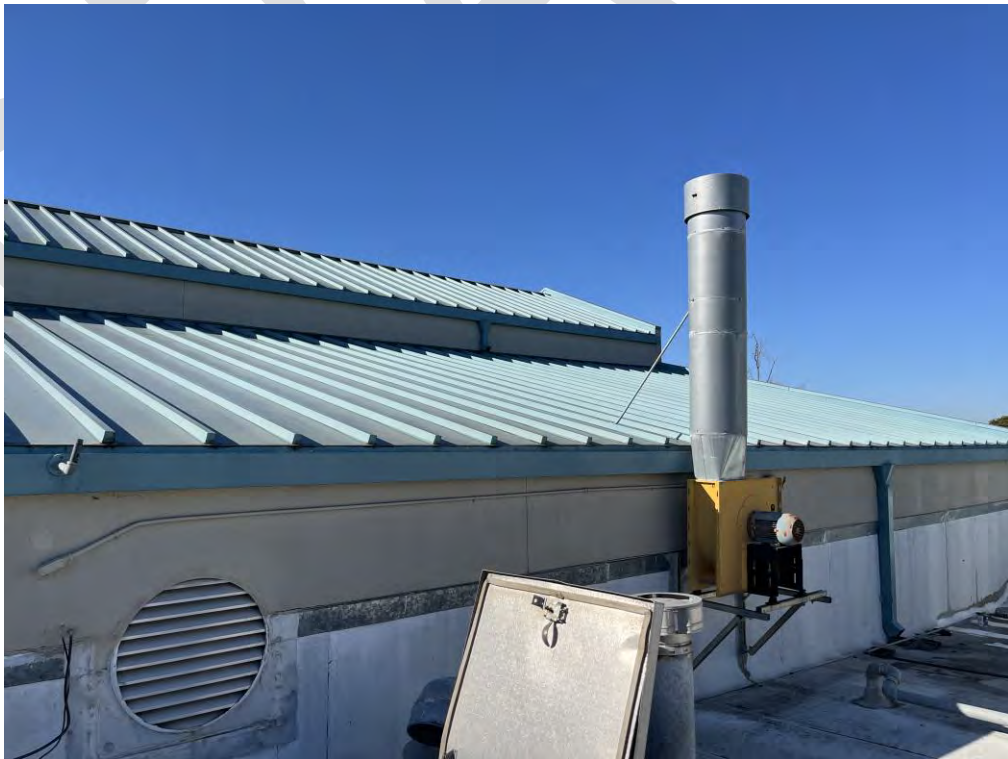
Photo 8: Roof of Apparatus Bay
