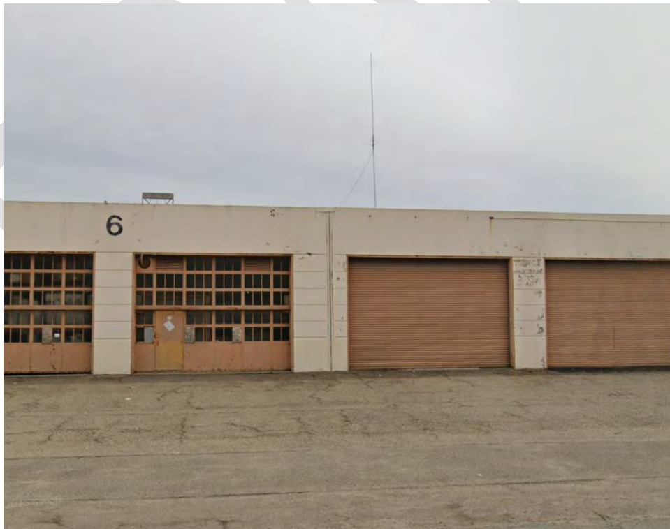
Photo 4: Western Face of Building at Seismic Gap
